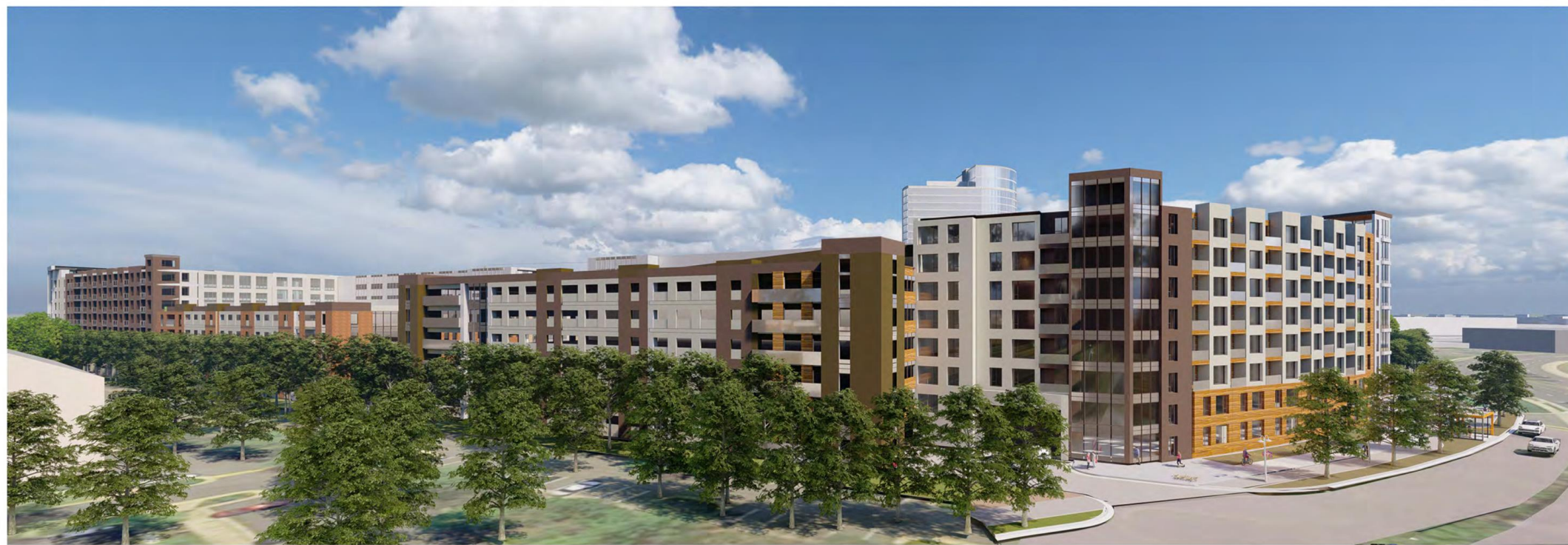
3 VIEW FROM NORTH WEST CORNER
