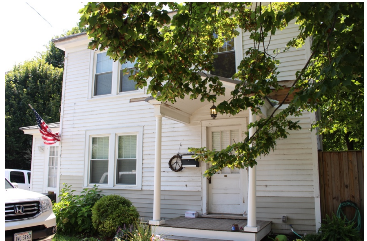
Photograph - Secondary Elevations or Details
