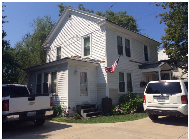
Photograph - Primary Elevation(s)
