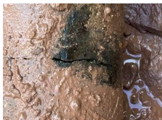
water main break
