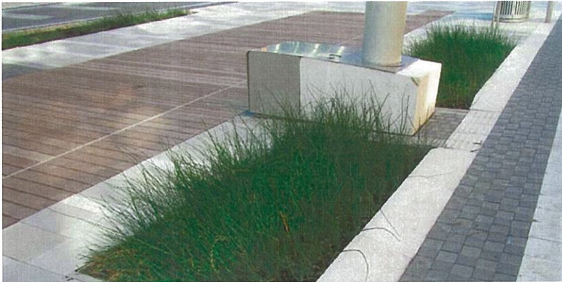
street verge stormwater catchment area with adjacent below grade storage
