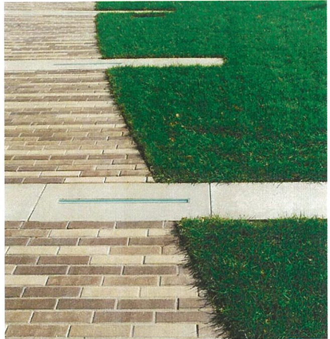
Decorative paving with integrated LED lighting
