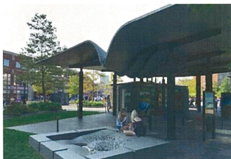
Artful canopy and stormwater collection
