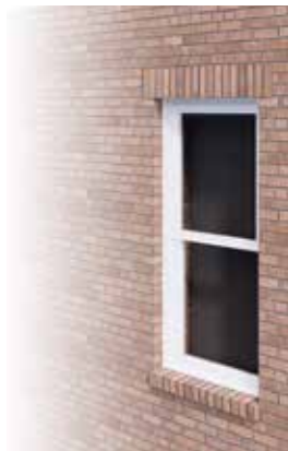
Brick lintels can be as simple as a single soldier course supported by a steel lintel behind. Other appropriate brick lintels include arches and jack arches. Brick sills are typically a single sloped rowlock.
