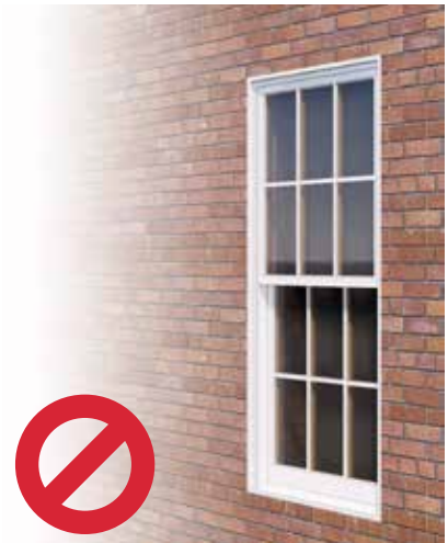
Flush Framing- Not Recommended
