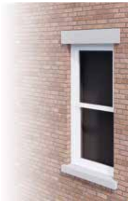
Brick lintel and sill made of stone, cast stone, concrete, or wood. Lintels should extend at least 4" beyond the edge of the masonry opening.
