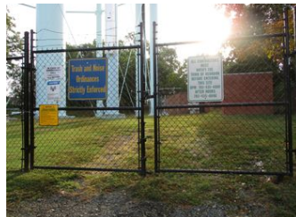
Spring Knoll Tank Site
