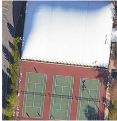
Bready Tennis Air Structure
