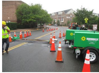
sample work zone
