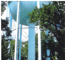
3rd Street Tank Site
