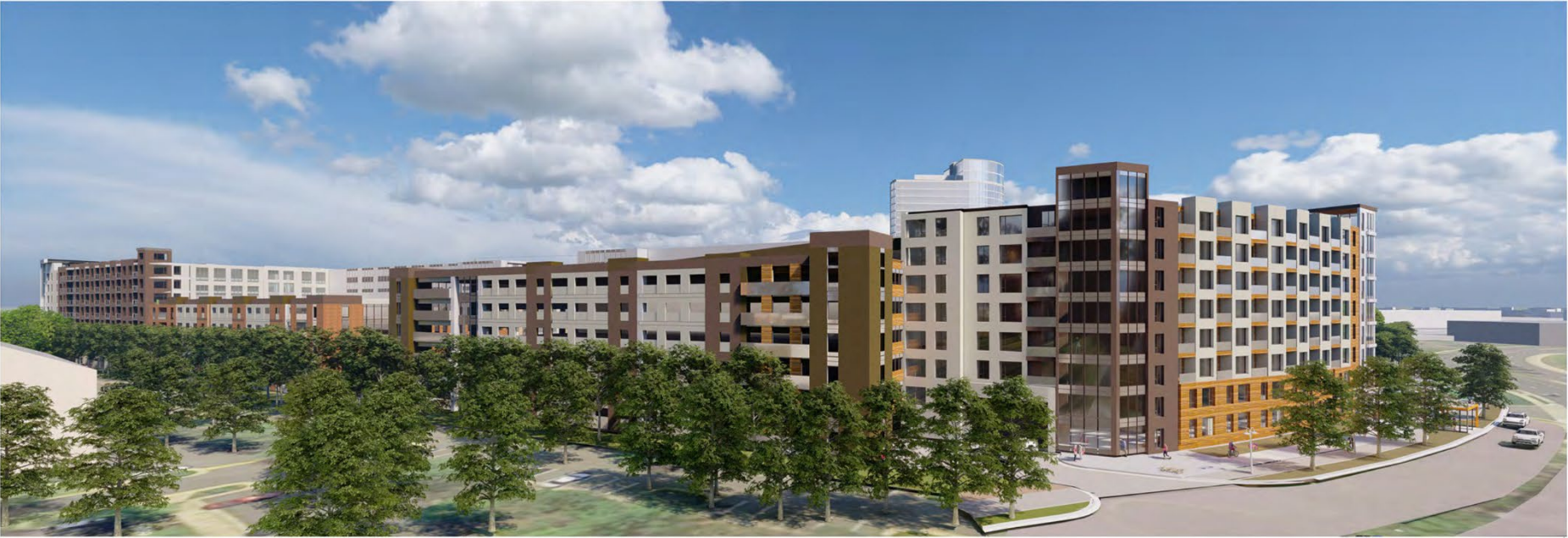
3 VIEW FROM NORTH WEST CORNER
