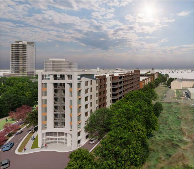
2 VIEW FROM NORTH EAST CORNER
