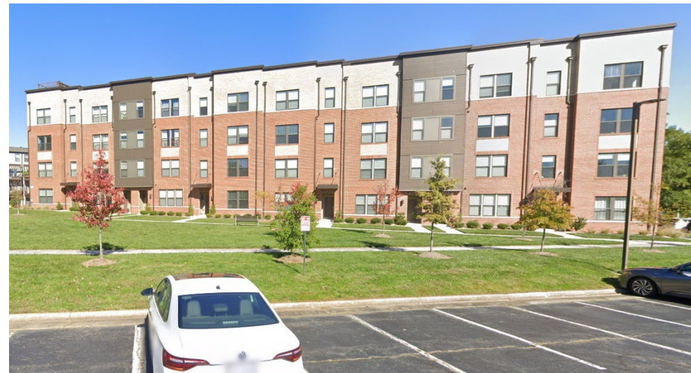
Metro Square Condominium Complex- Town of Herndon, VA
