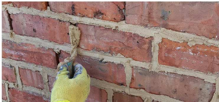
Repointing masonry. Image Credit: TurnBullMasonry.com
