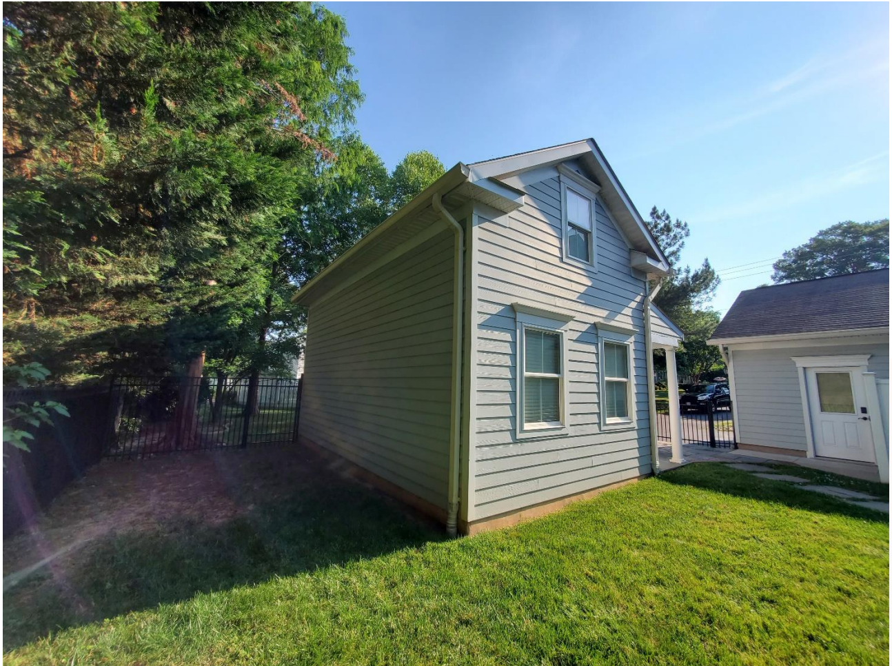
Rear of Garage
