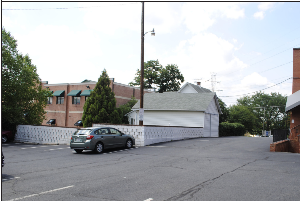
EXIST BUILDING TO RIGHT (WEST) OF MAIN BUILDING
