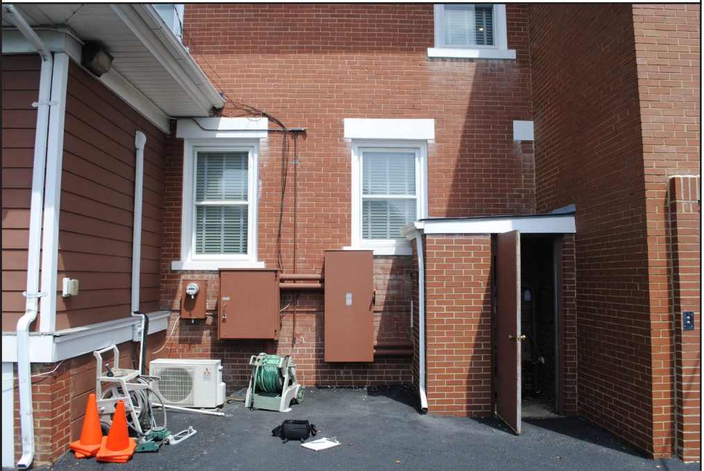
EXIST ELEVATOR CONTROL ROOM
