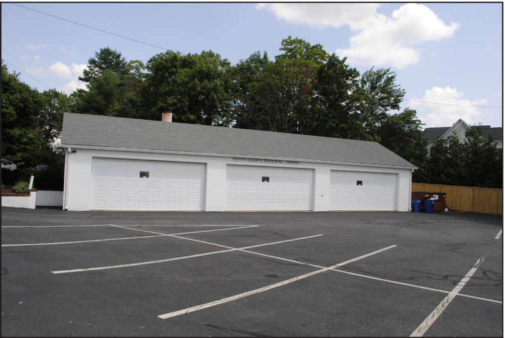
EXIST GARAGE TO SOUTH EAST OF EXIST BUILDING
