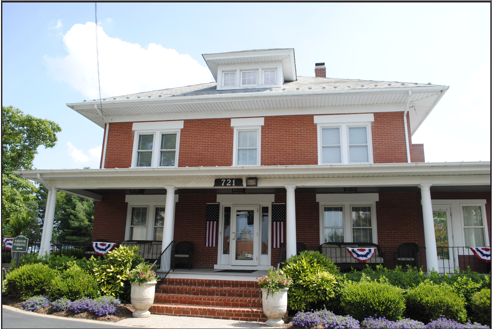
EXIST BUILDING FRONT (NORTH) ELEVATION
