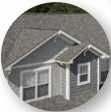
Roofing and Ventilation
