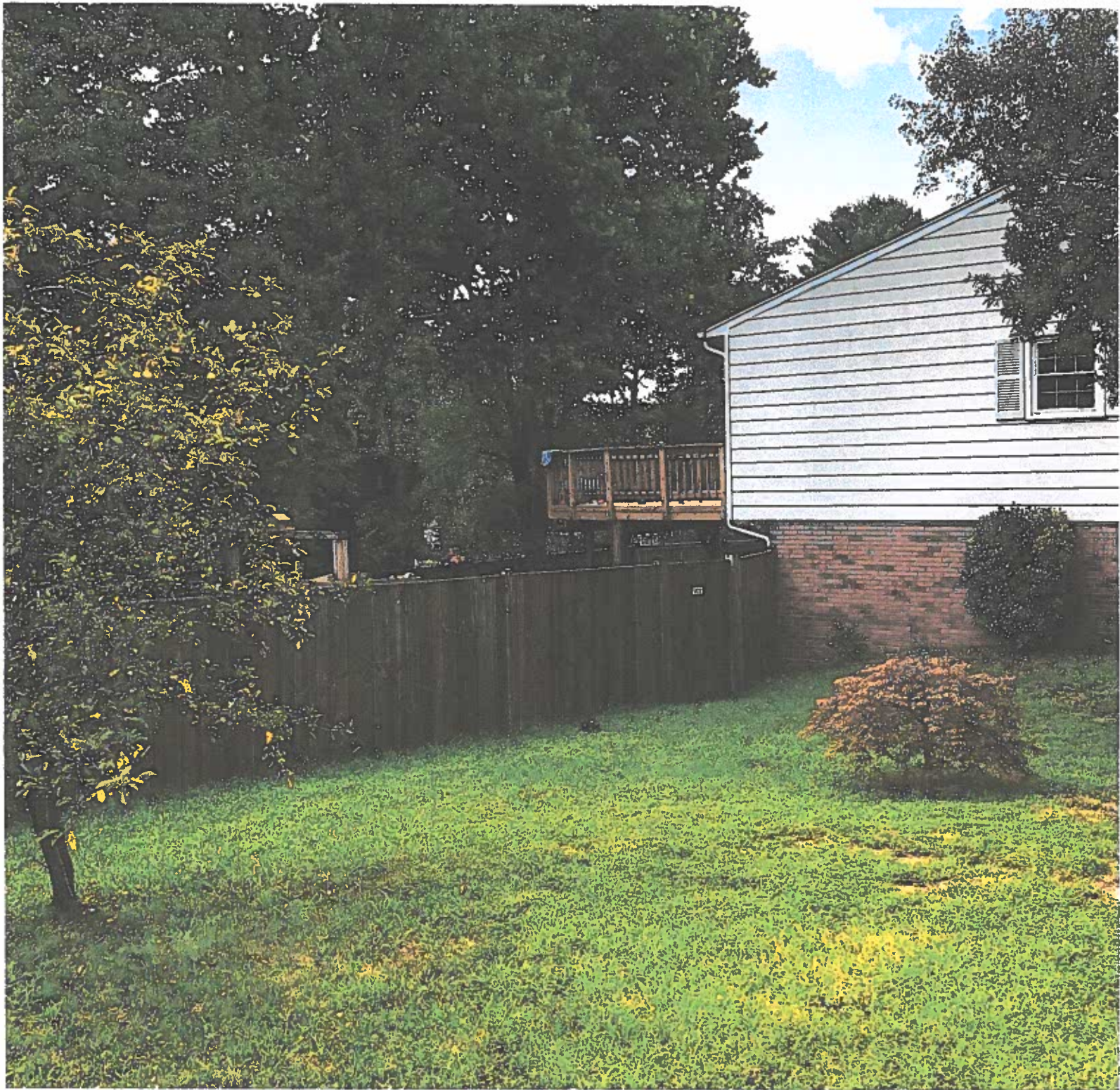
Sidewalk view of deck from side of house oppos of proposed stairs addition
