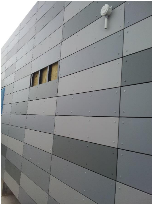
Figure 1 Example rainscreen exterior wall system
