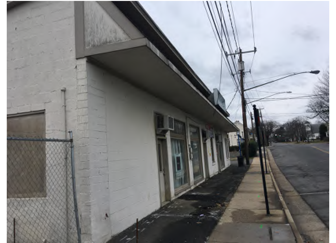
Neighboring Structure to the West
