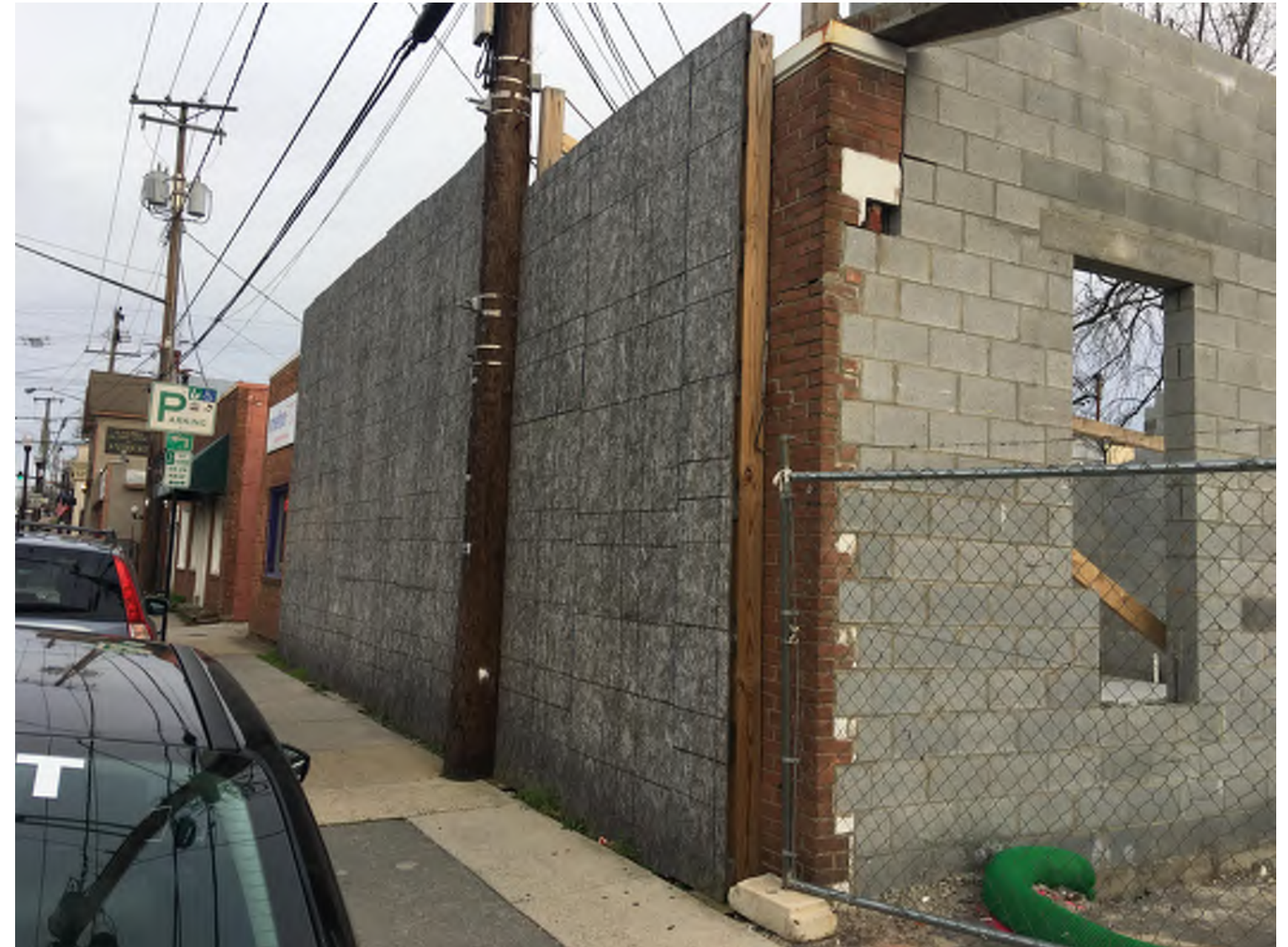
North Elevation, Looking Westerly
