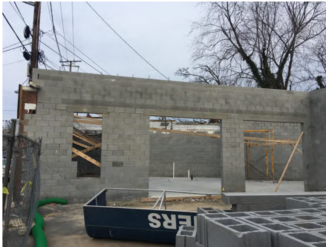
West Elevation, North End
