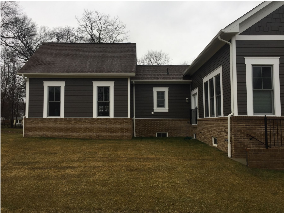
719 Dranesville Road South side of house
