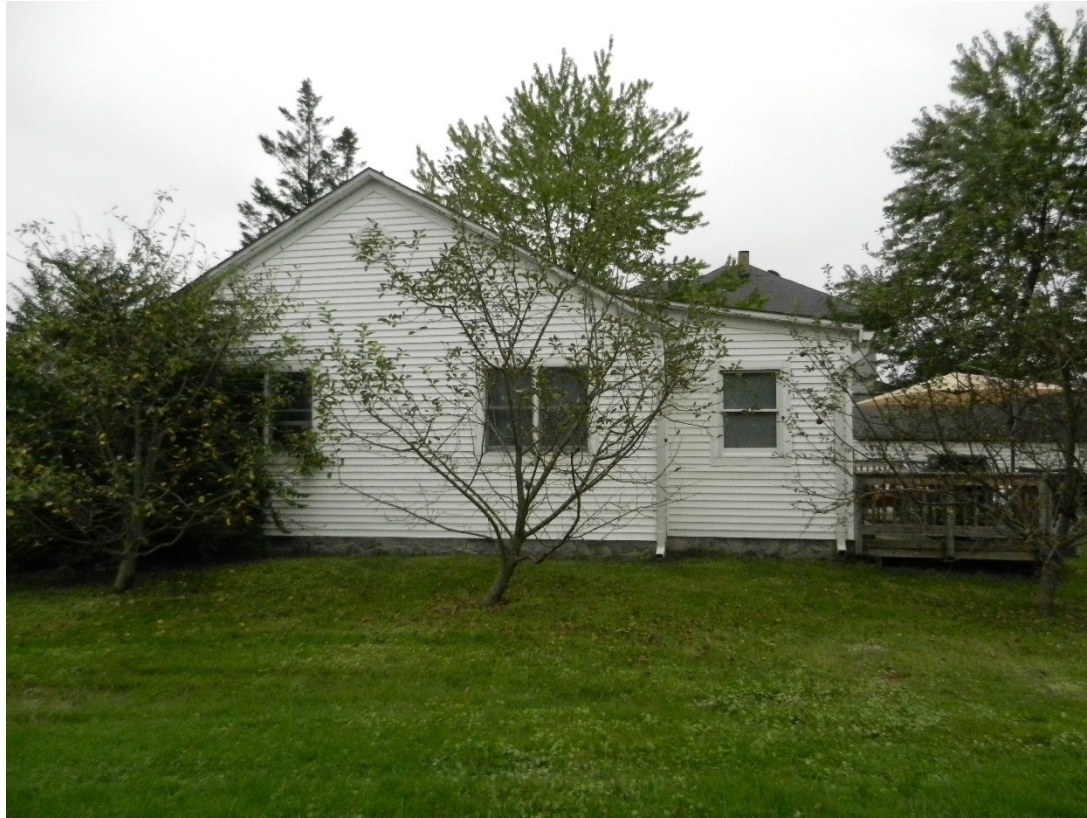
Right side, neighboring lot (641 Nash St. / Spring Street) facing
