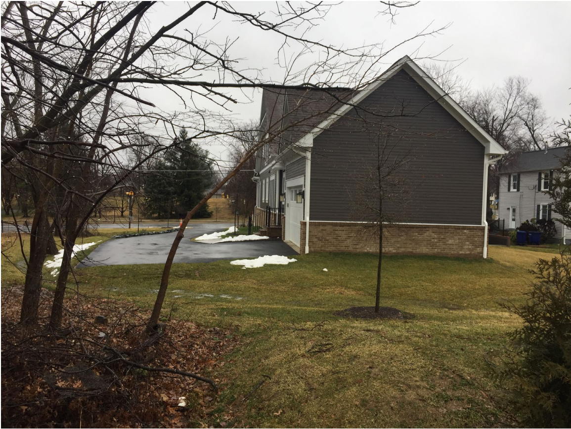
719 Dranesville Road Northwest side of house
