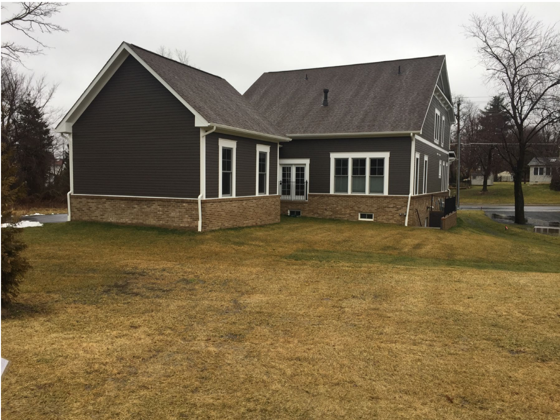
719 Dranesville Road West side of the house
