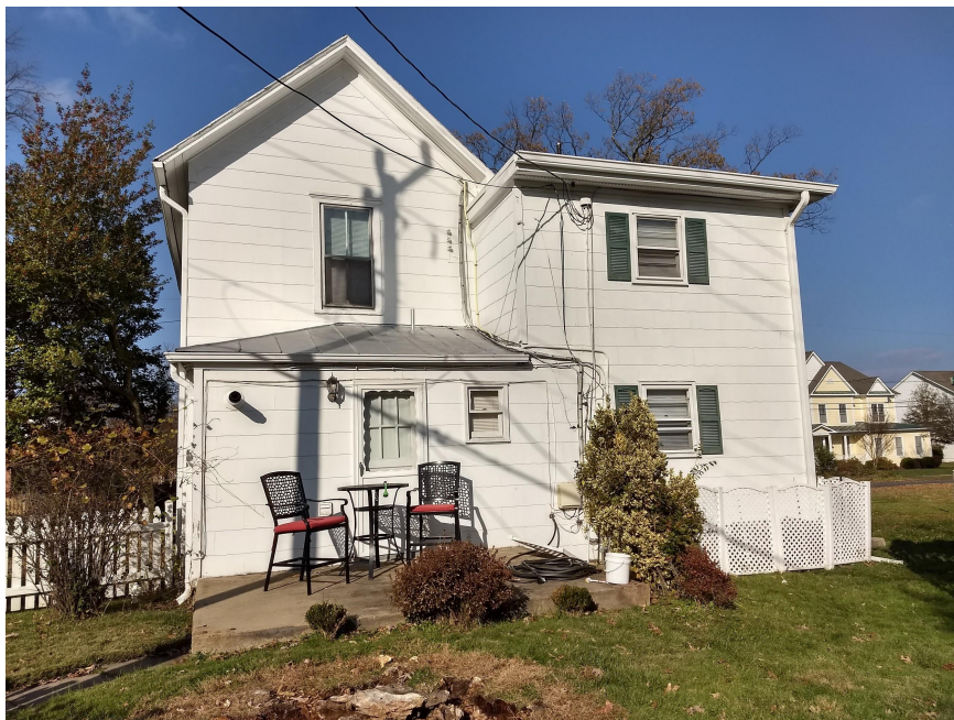
Rear North Side
