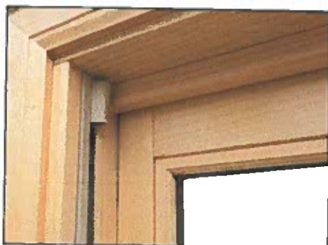
Wood Parting Stop, Concealed Jambliner
