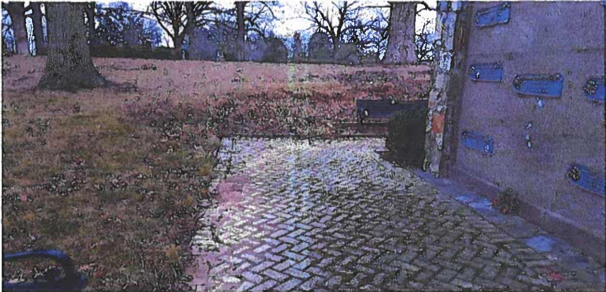
Mausoleum # 2 West side.
