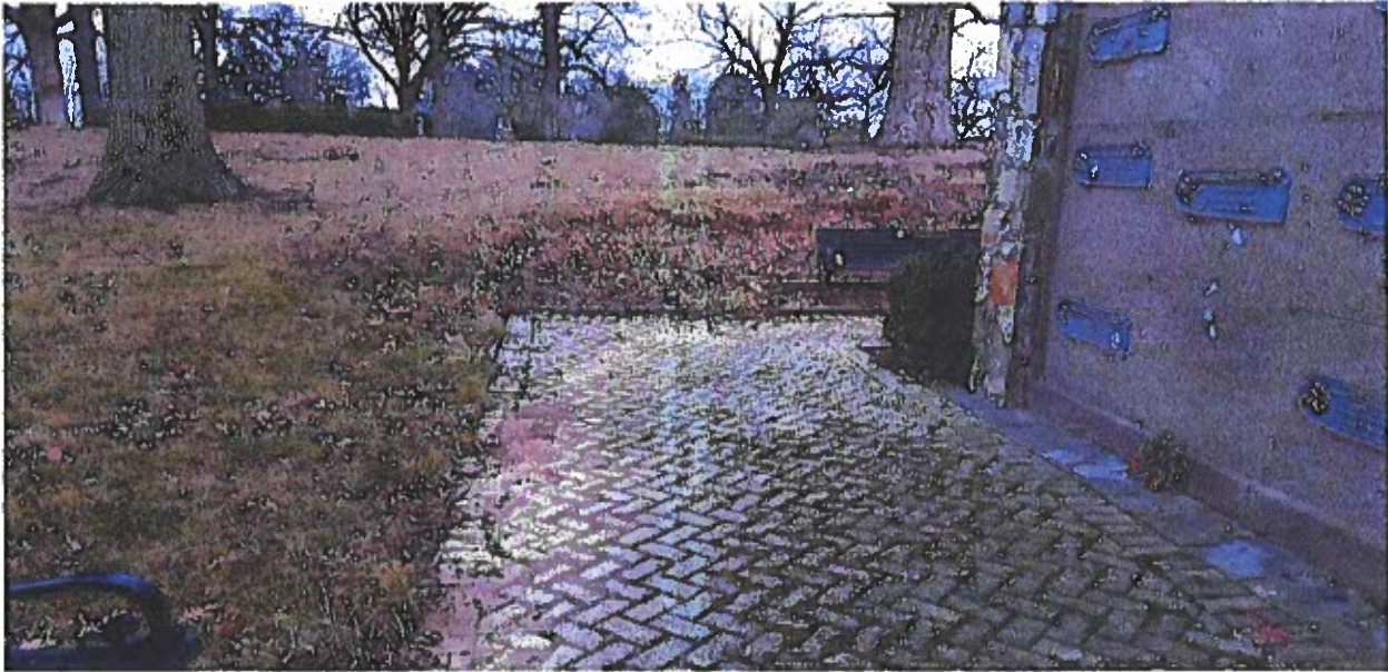
Mausoleum # 2 West side.
