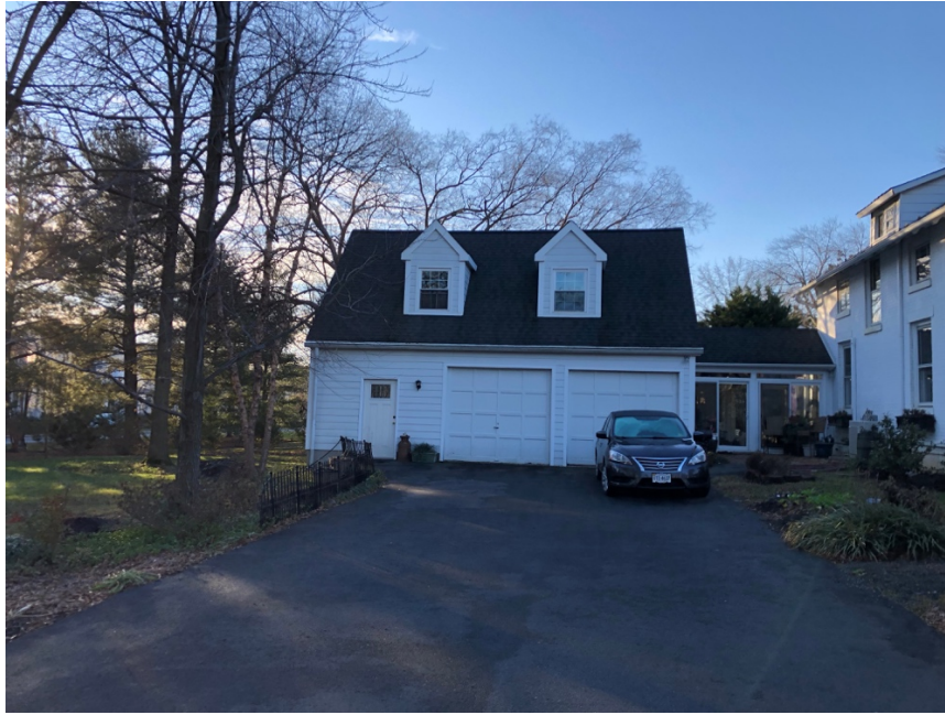
Garage front elevation. (note existing garage doors)
