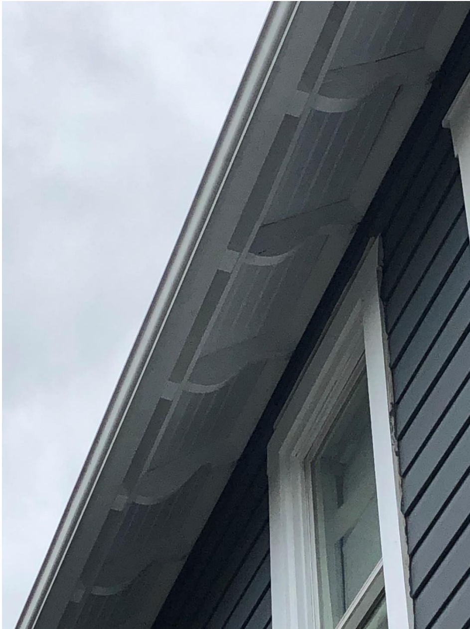
DETAIL OF EXISTING HOUSE'S RAFTER TAILS
