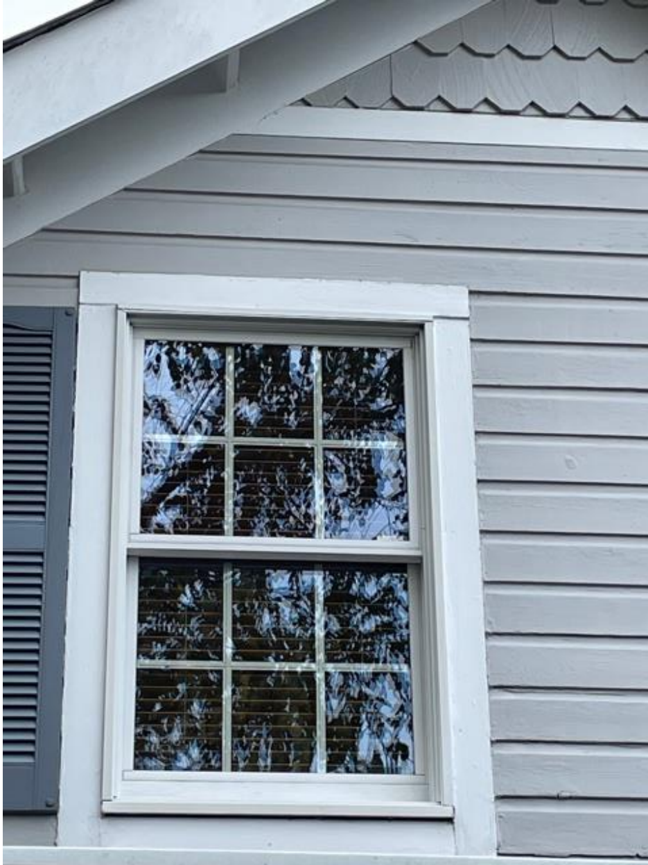
Existing Window and Trim
