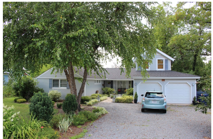
Photograph - Primary Elevation(s)
