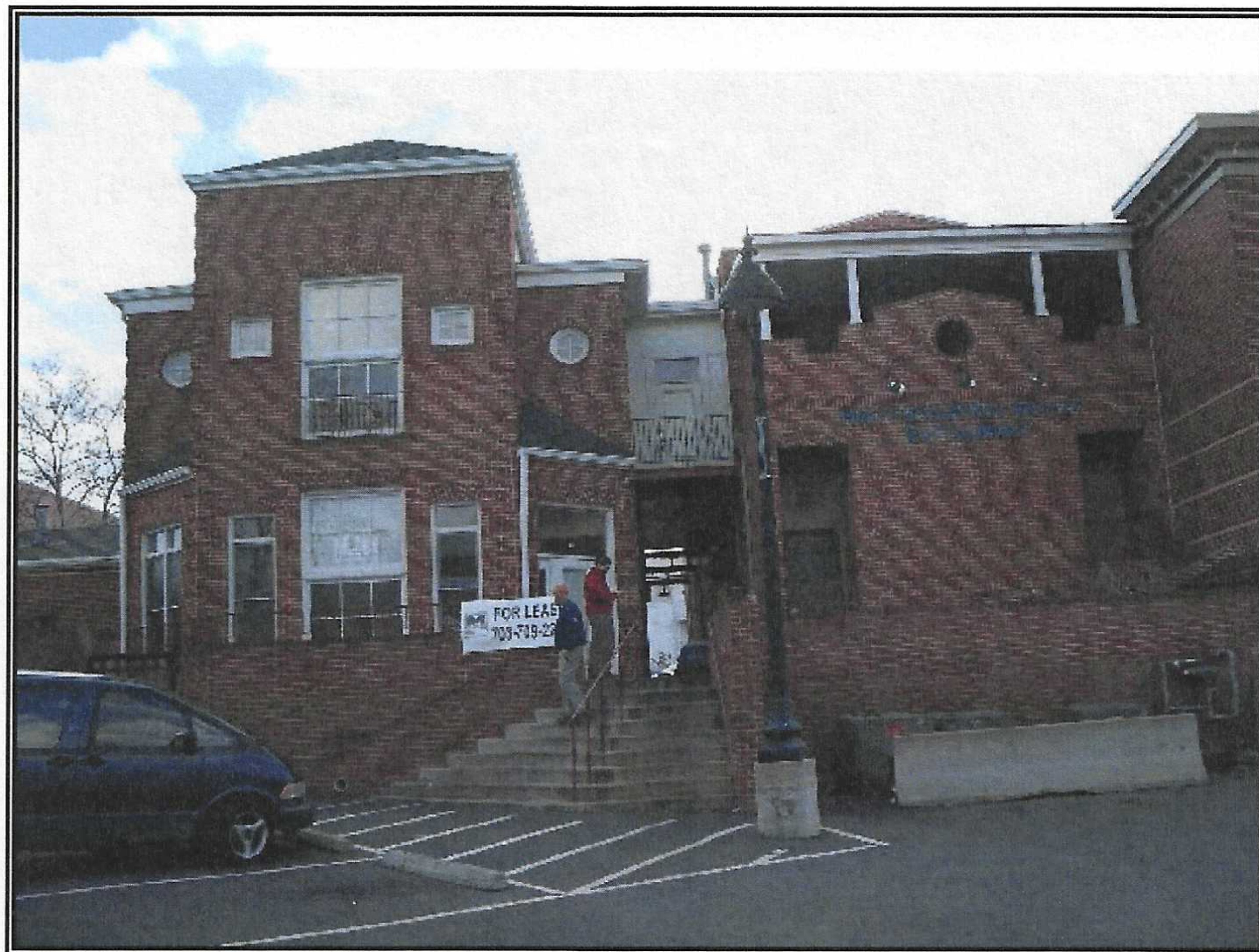
Rear of subject property.
