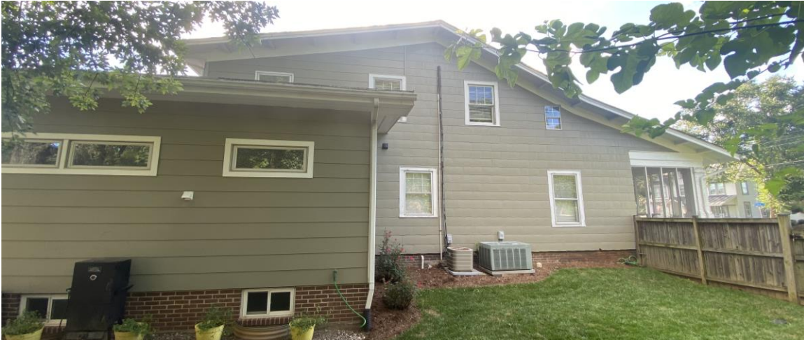
Left Façade- Looking toward Spruce Street
