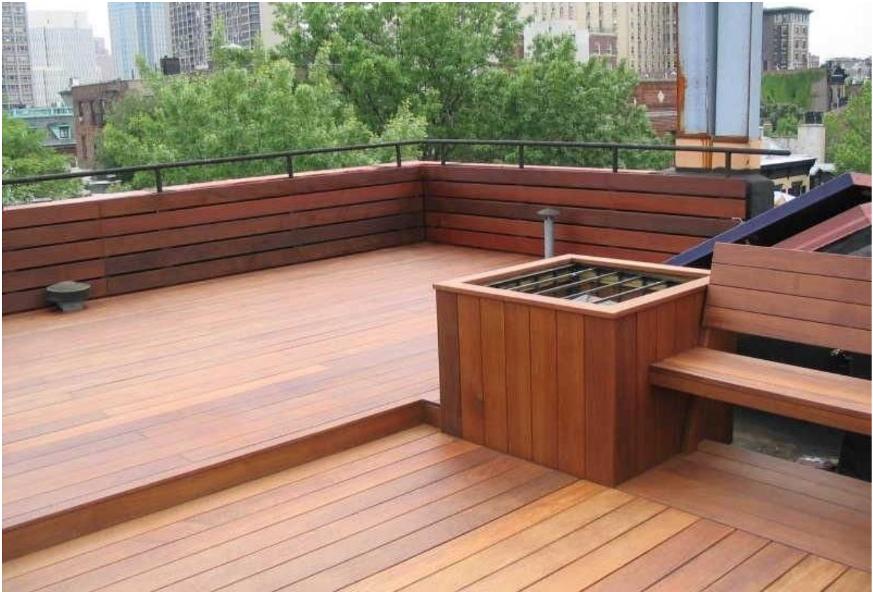
Idea for revised design – split solution with shorter solid wall and open railing
