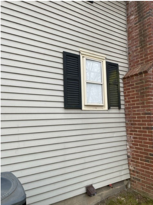
4. Bathroom Window: Side of house
