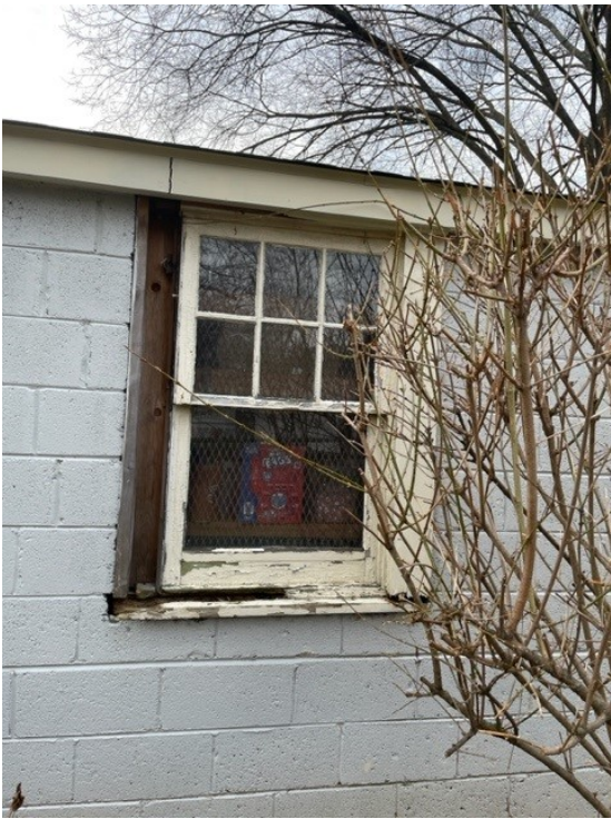
5. Garage Window: Left Side.
