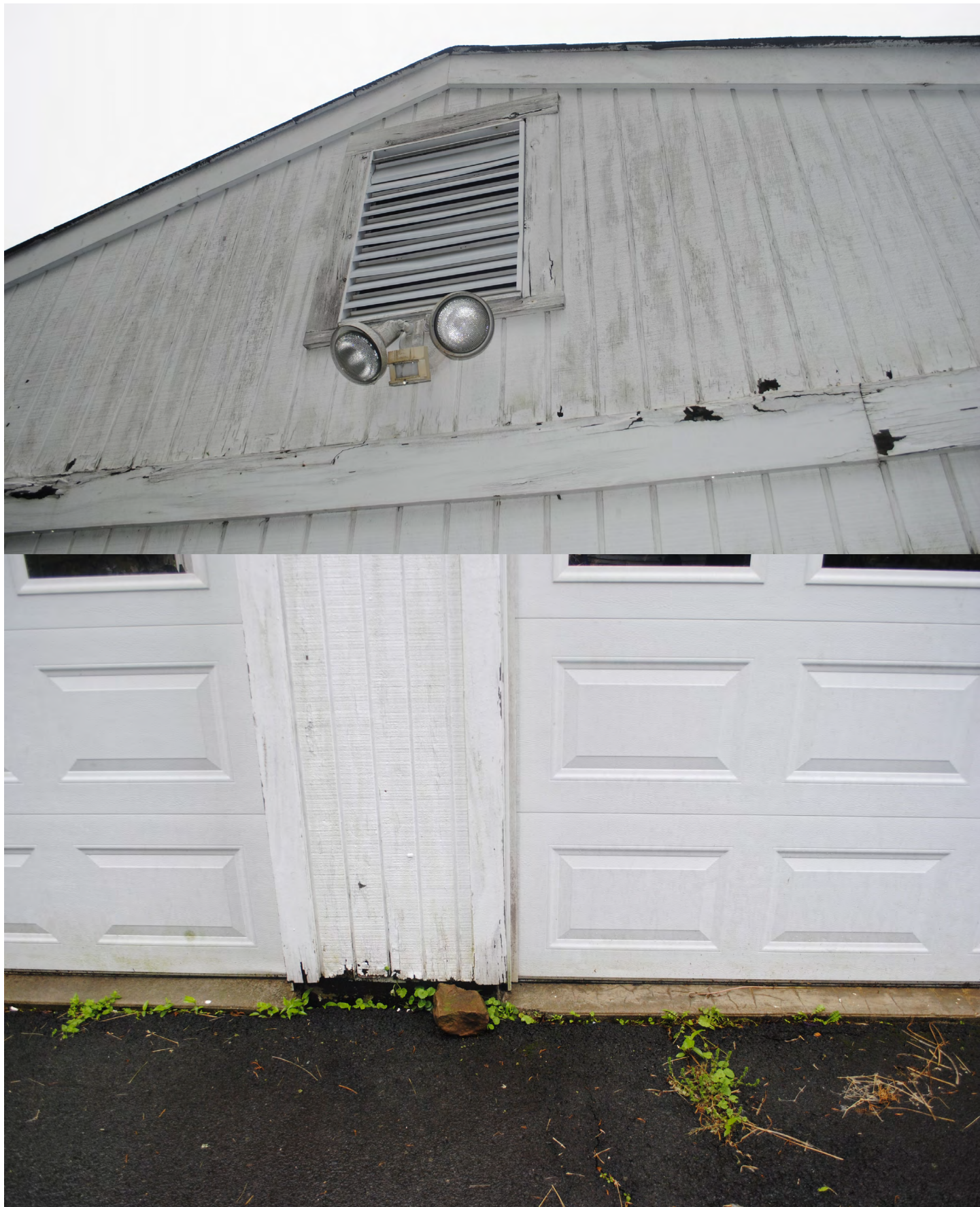
EXISTING GARAGE CONDITION
