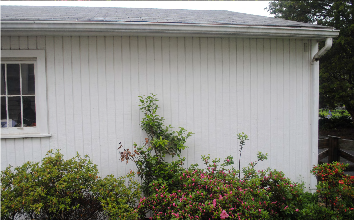
EXISTING GARAGE, LEFT ELEVATION
