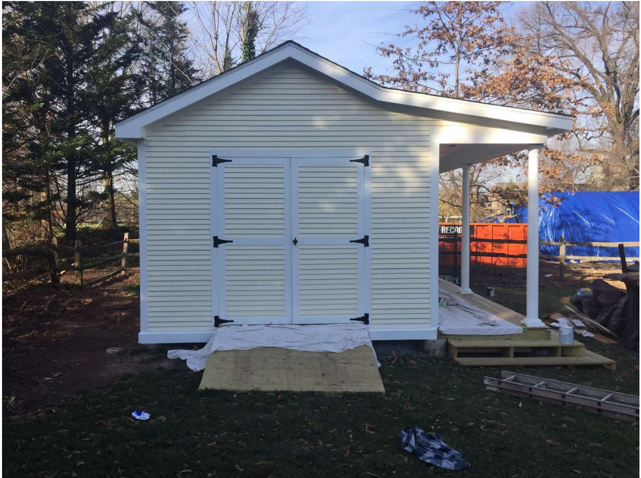
Shed Side (South Elevation):
