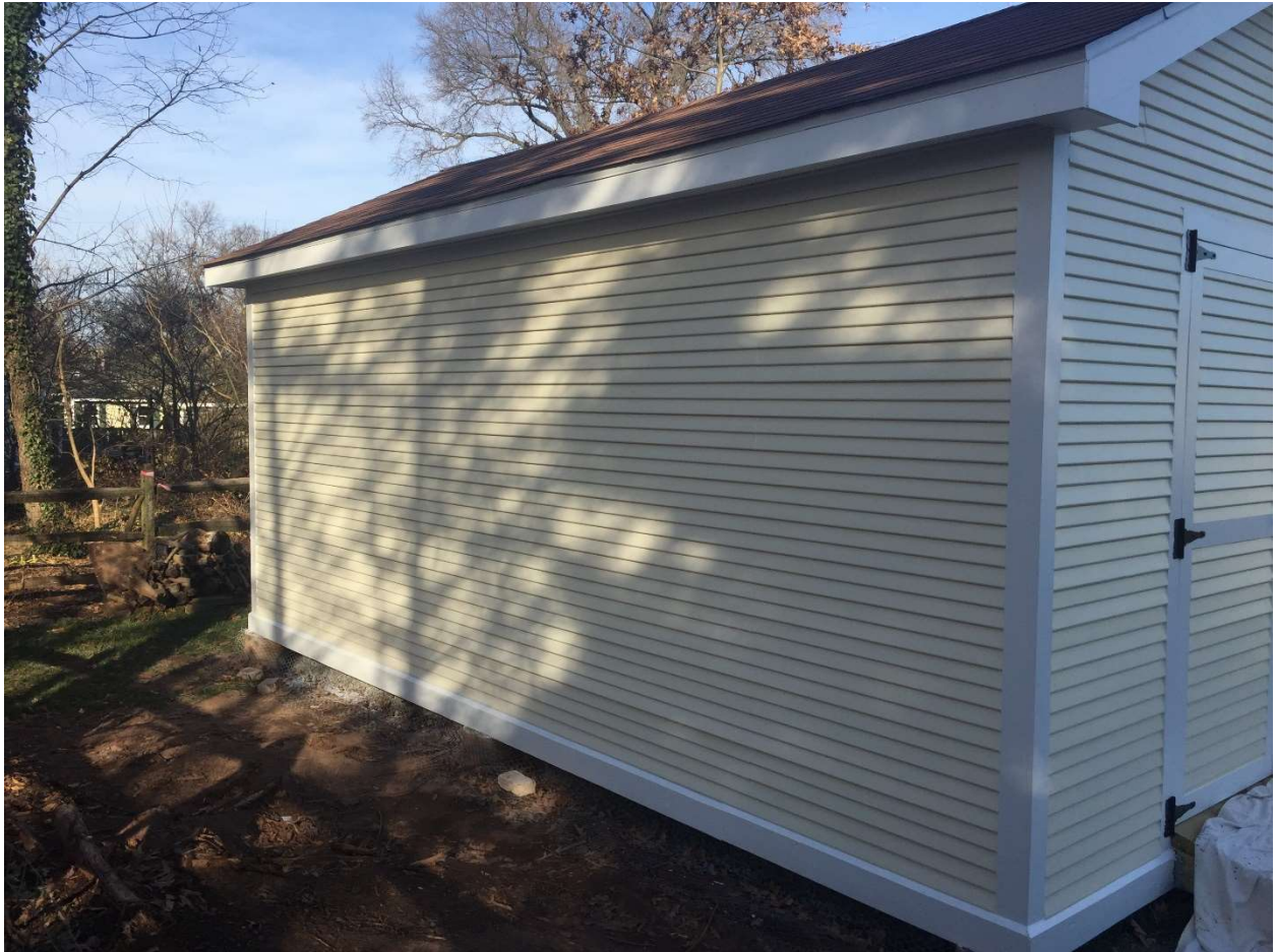
Shed Rear (West Elevation):
