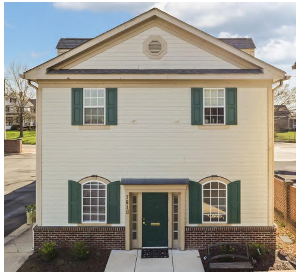
EXISTING PICTURE OF 761B
