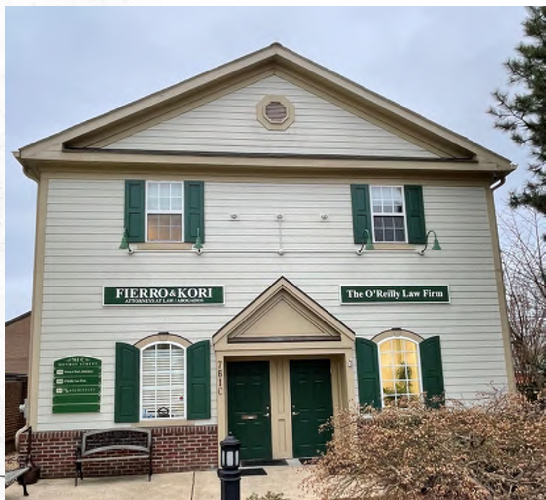
EXISTING PICTURE OF 761C
