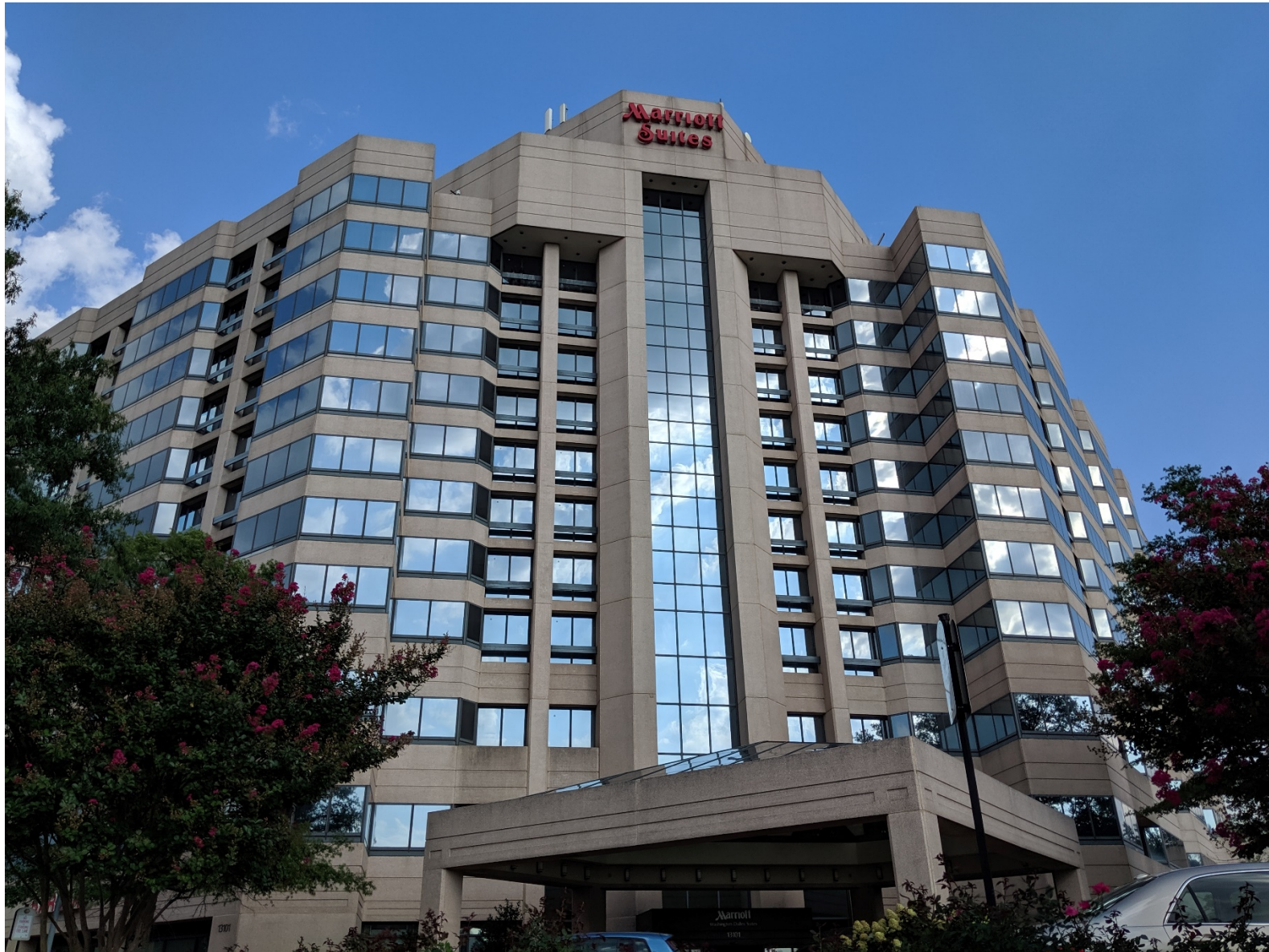
East Elevation Looking at Marriott Suites
