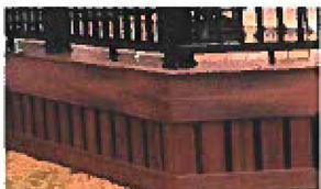
2 WOOD DECKING EDGE, TREATED WOOD, COLOR TBD
