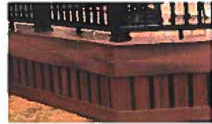
2 WOOD DECKING EDGE TREATED WOOD, COLOR TBD
