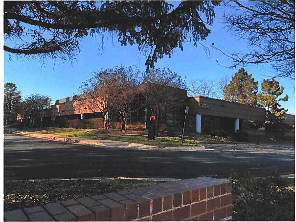
SPRINGPARK - BUILDING 455 EXISTING SITE IMAGES
