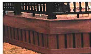
2 WOOD DECKING EDGE, TREATED WOOD, COLOR TBD
