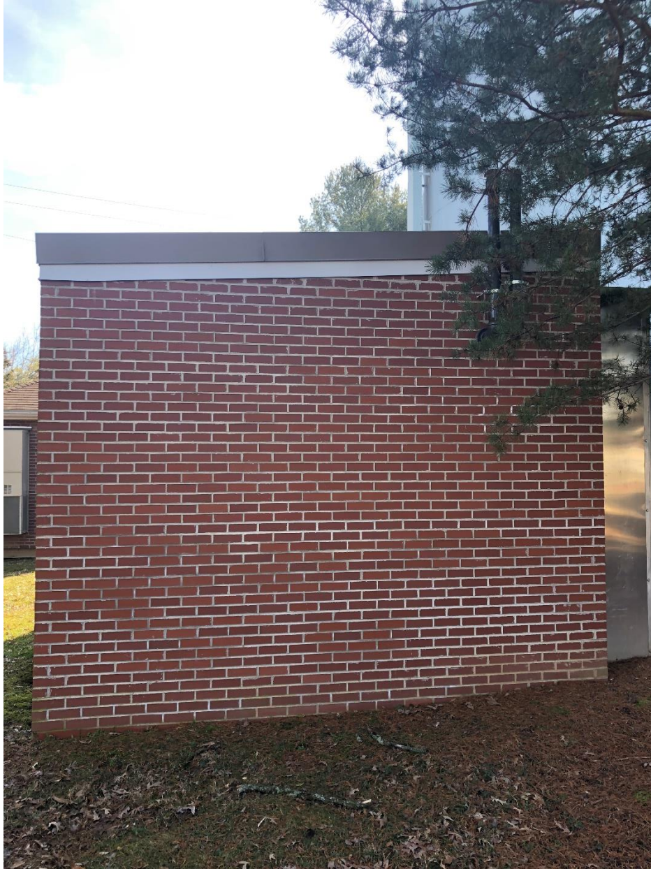
Verizon Generator Stealth Enclosure
