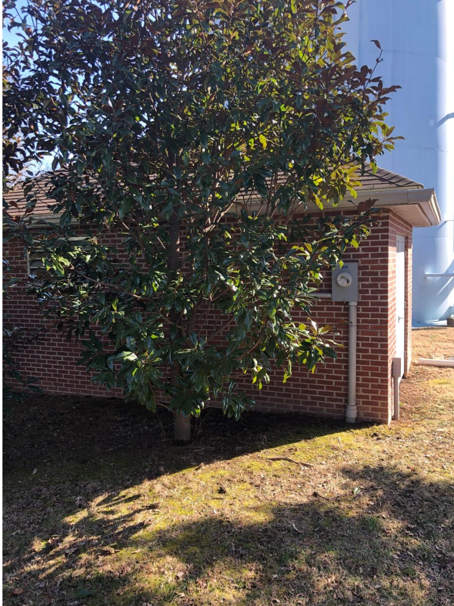
T-Mobile Equipment Shelter
