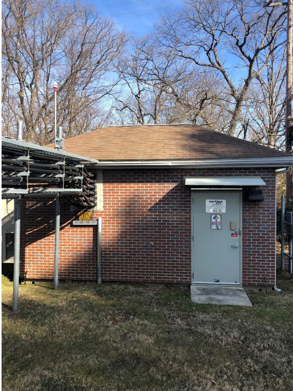
Verizon Equipment Shelter
