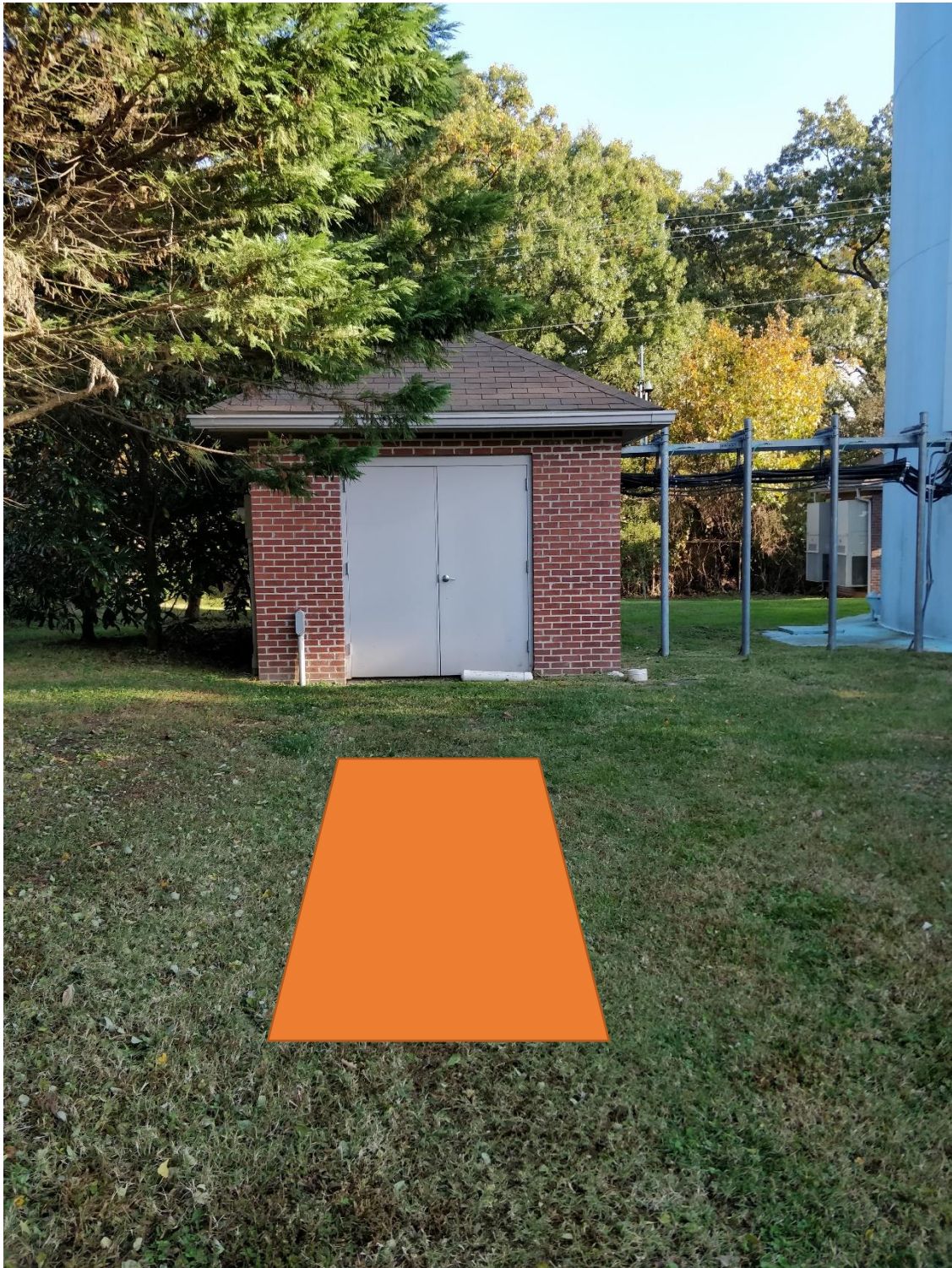
T-Mobile Equipment Shelter and Proposed Generator location
