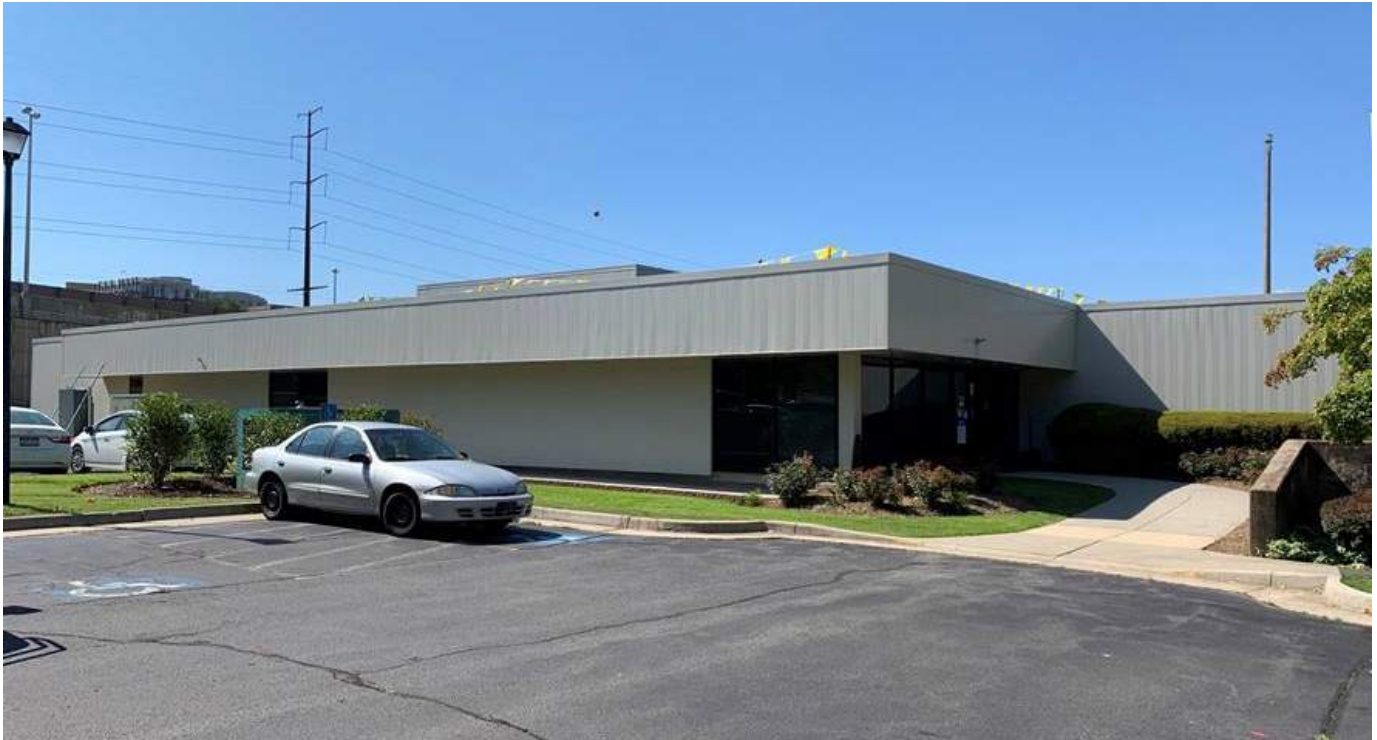
MAIN BUILDING – FRONT
