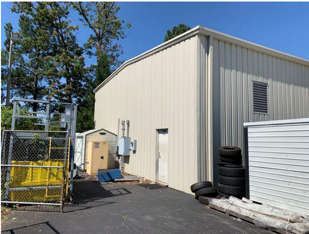
GARAGE – LEFT SIDE
