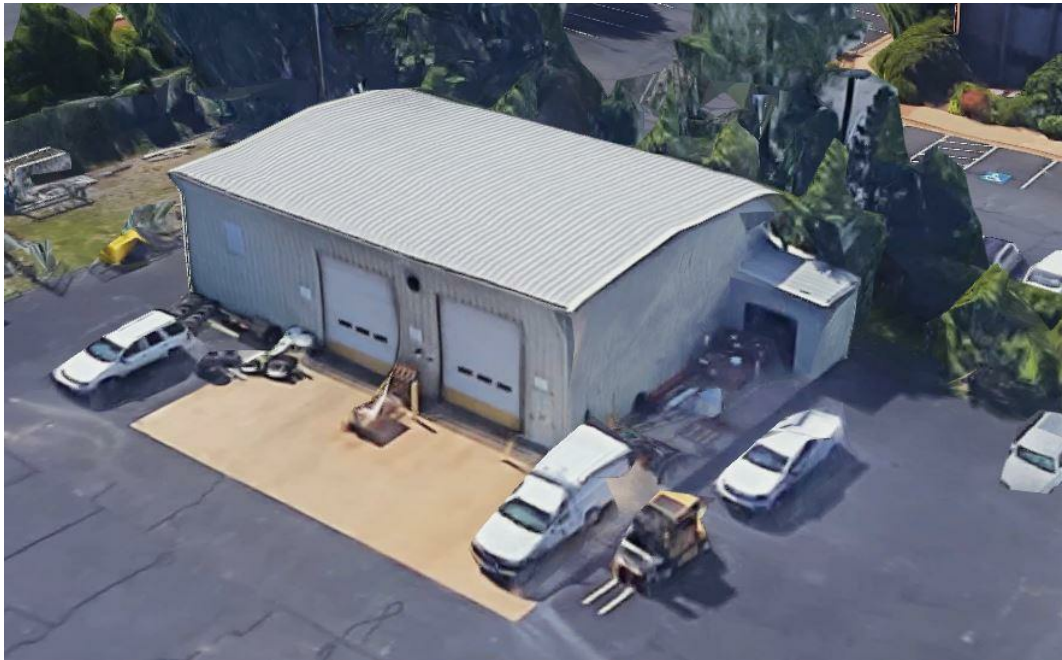
4 EXISTING VEHICLE GARAGE - Aerial View, Looking Southwest 1/2" = 1'-0"
