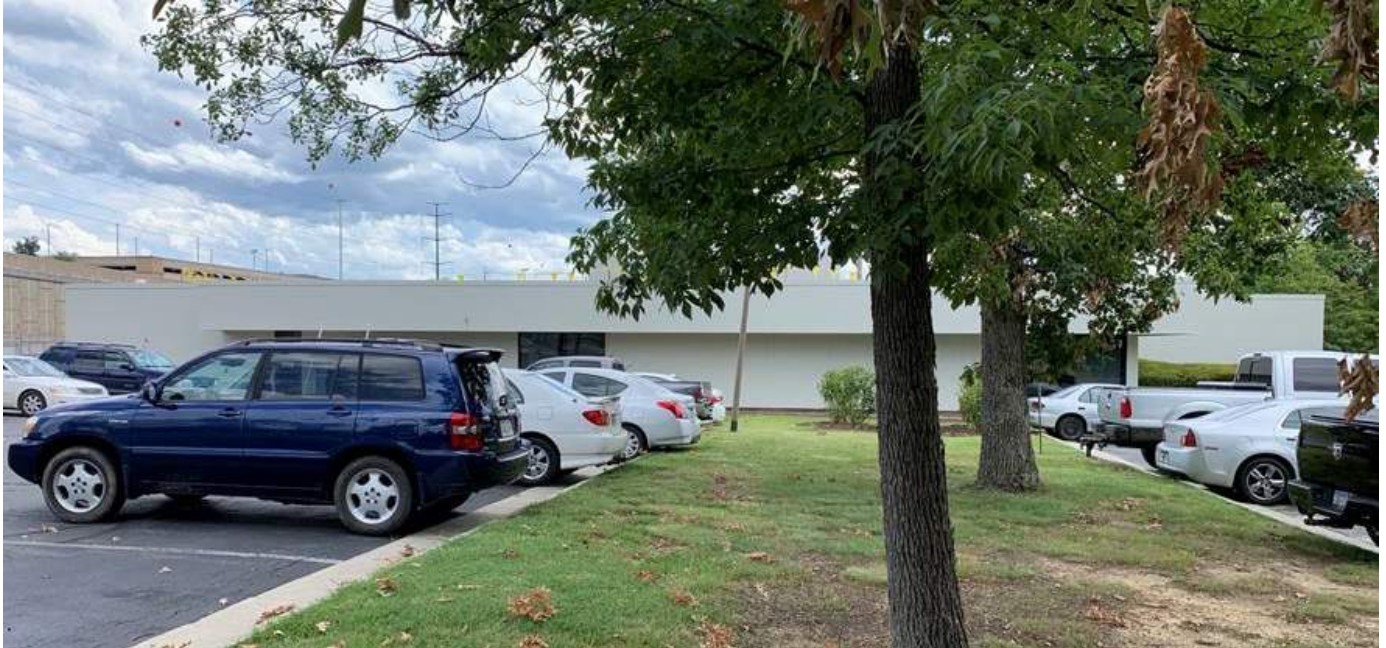
MAIN BUILDING – FRONT
