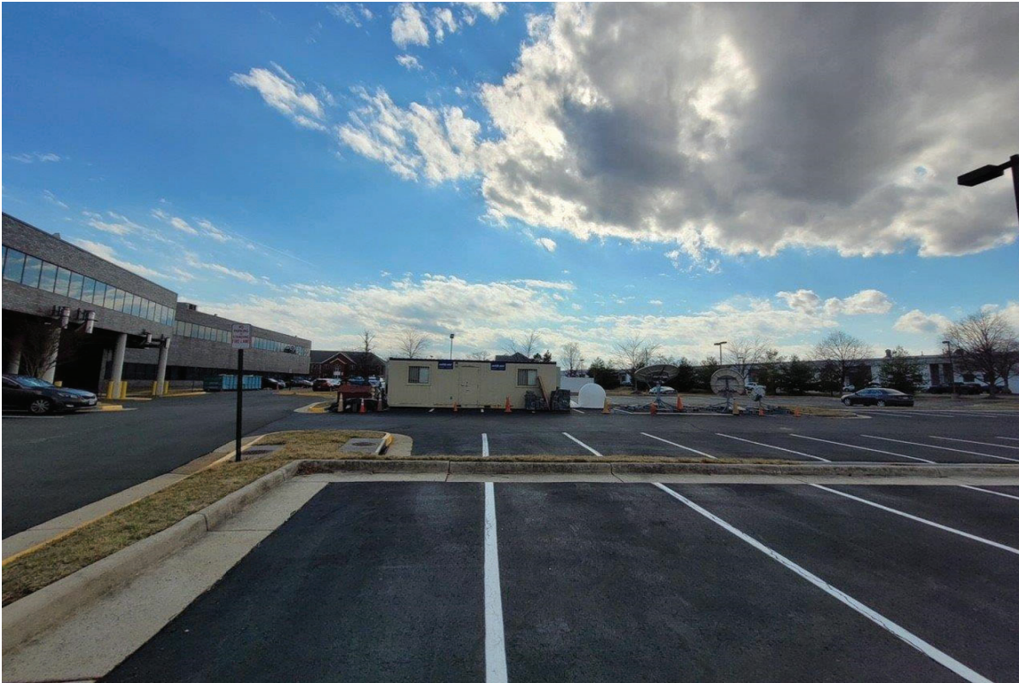
Existing North Storage Area
