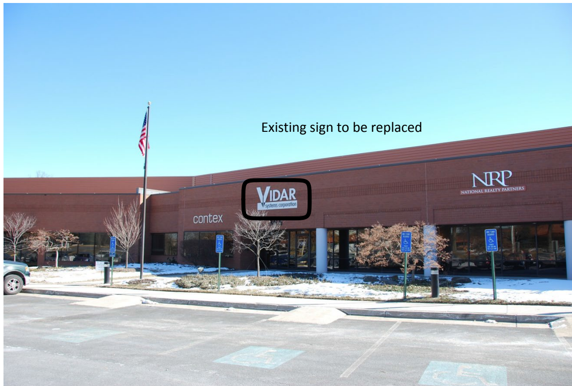
Exterior view front façade looking northeast
