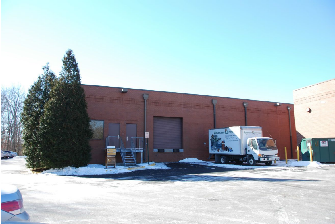
Exterior view of rear loading area
