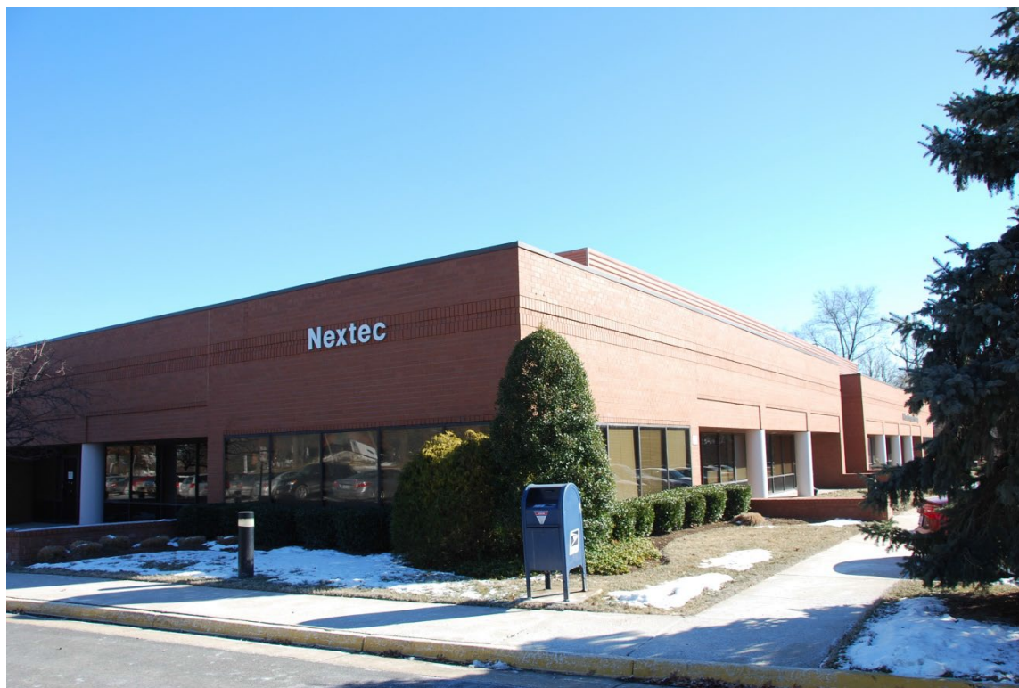
Exterior view of southern façade looking east
