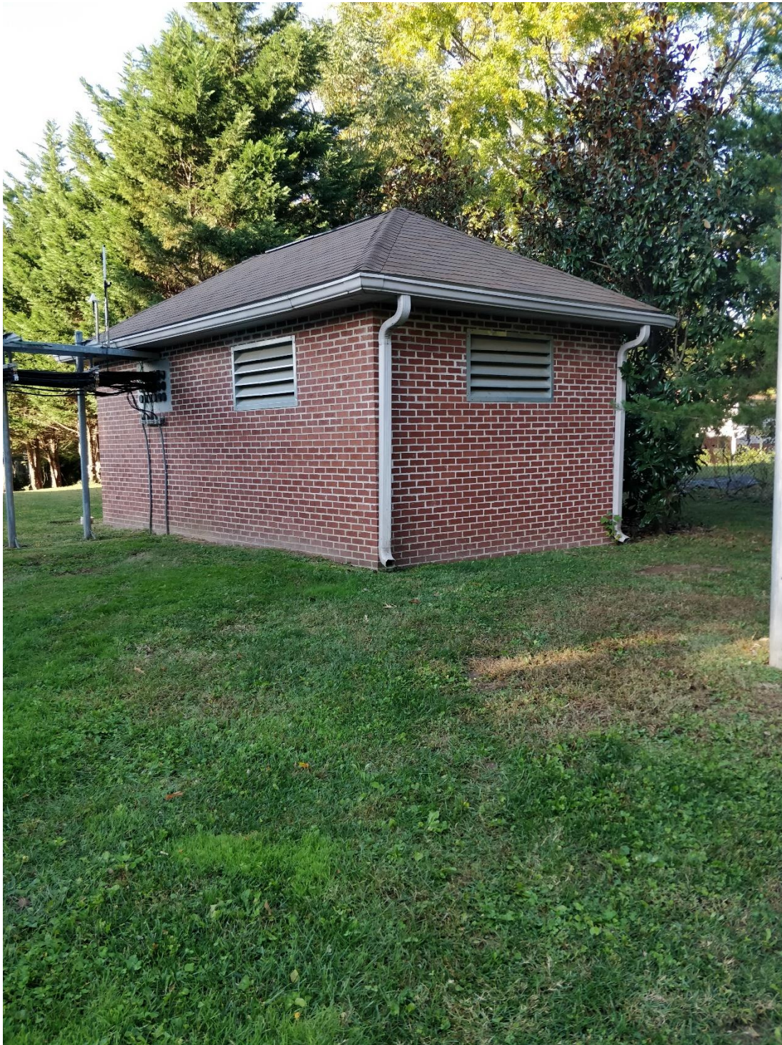
T-Mobile Equipment Shelter
