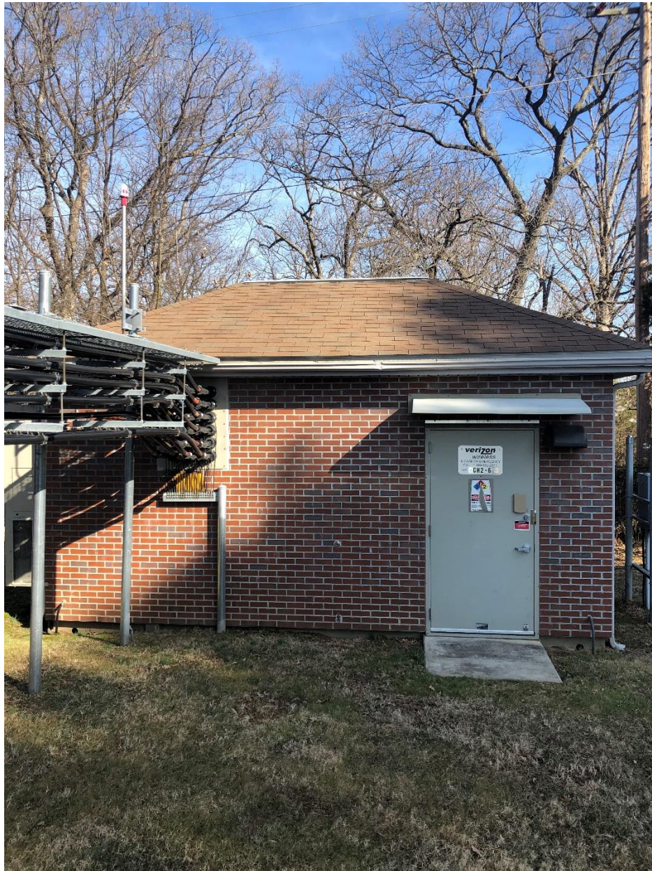
Verizon Equipment Shelter
