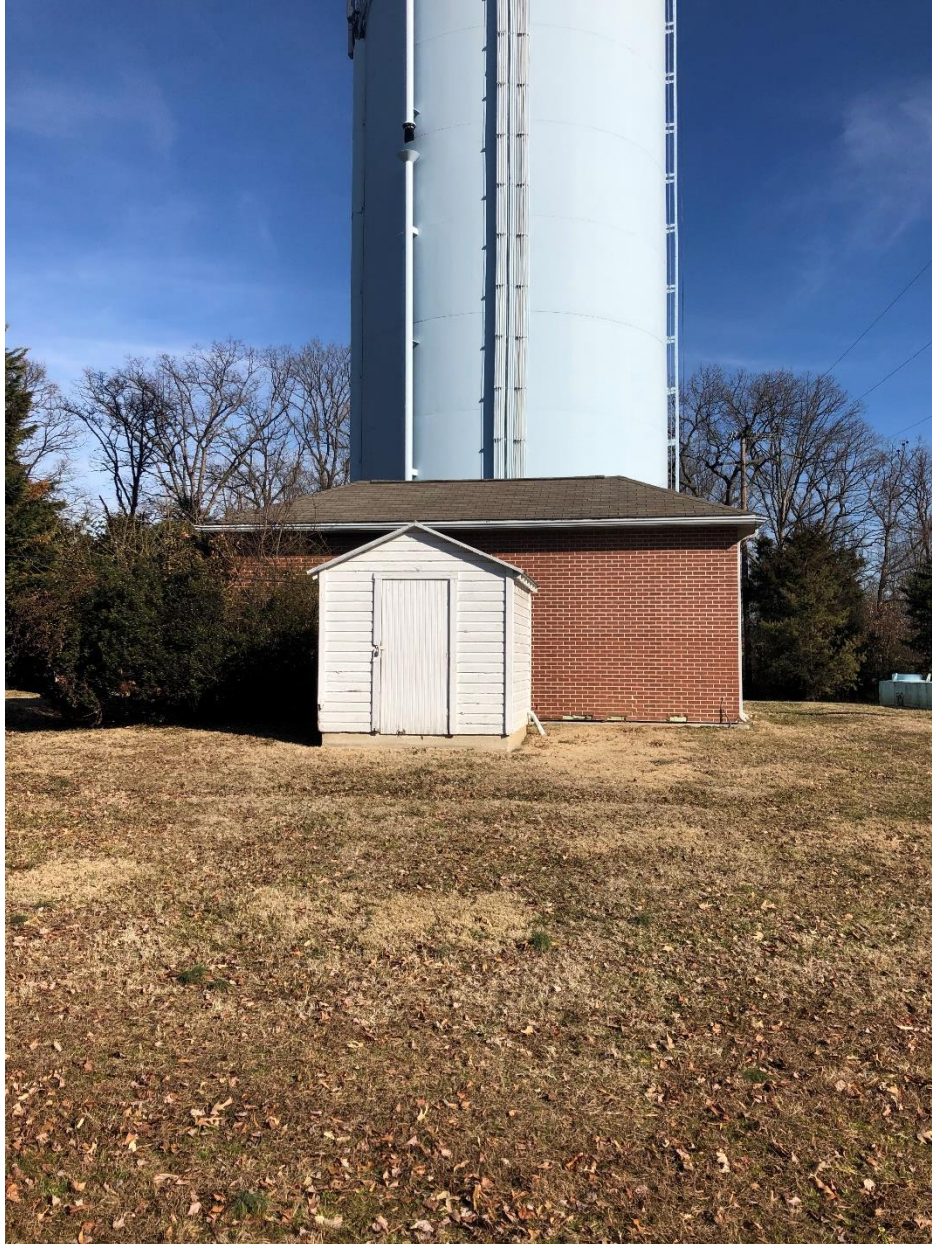
AT&T Equipment Shelter
