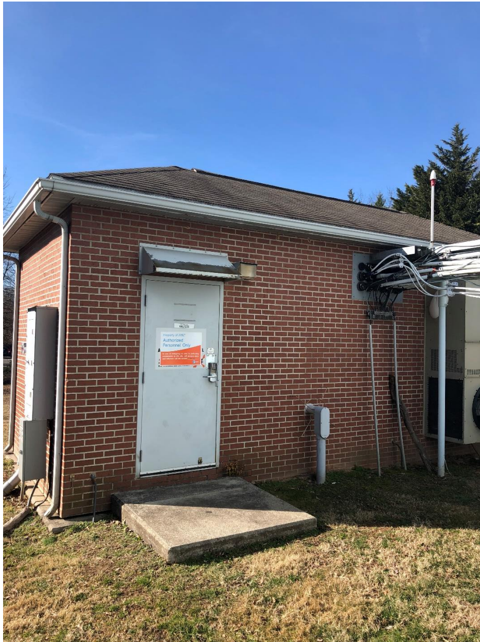
AT&T Equipment Shelter
