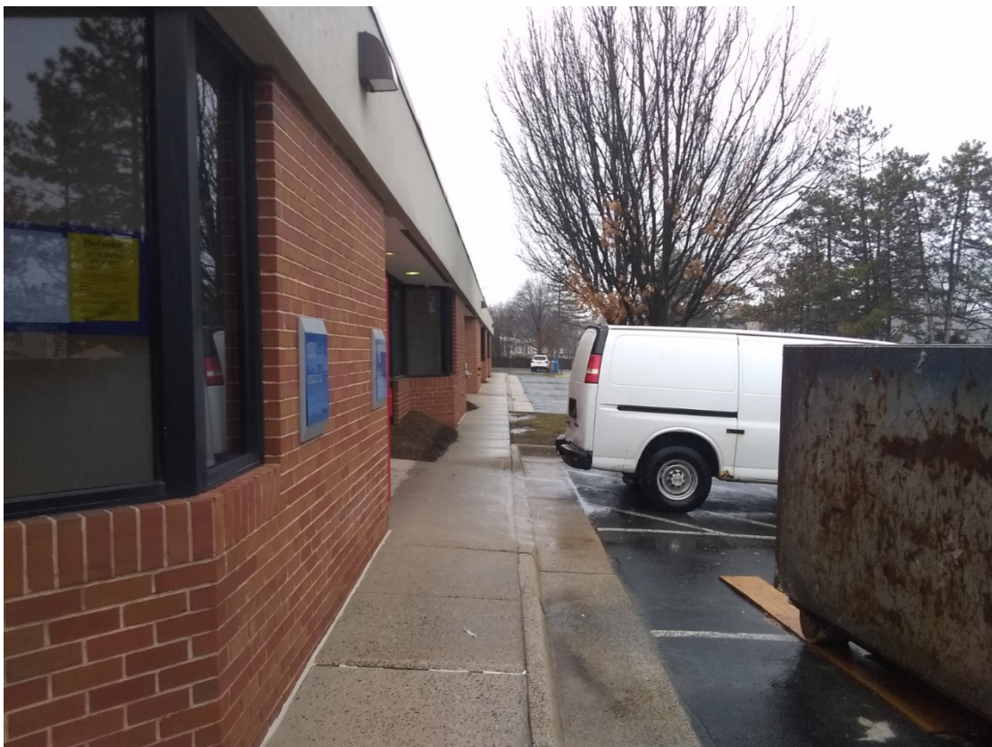
VIEW LOOKING SOUTHWEST ALONG BUILDING WEST ELEVATION
