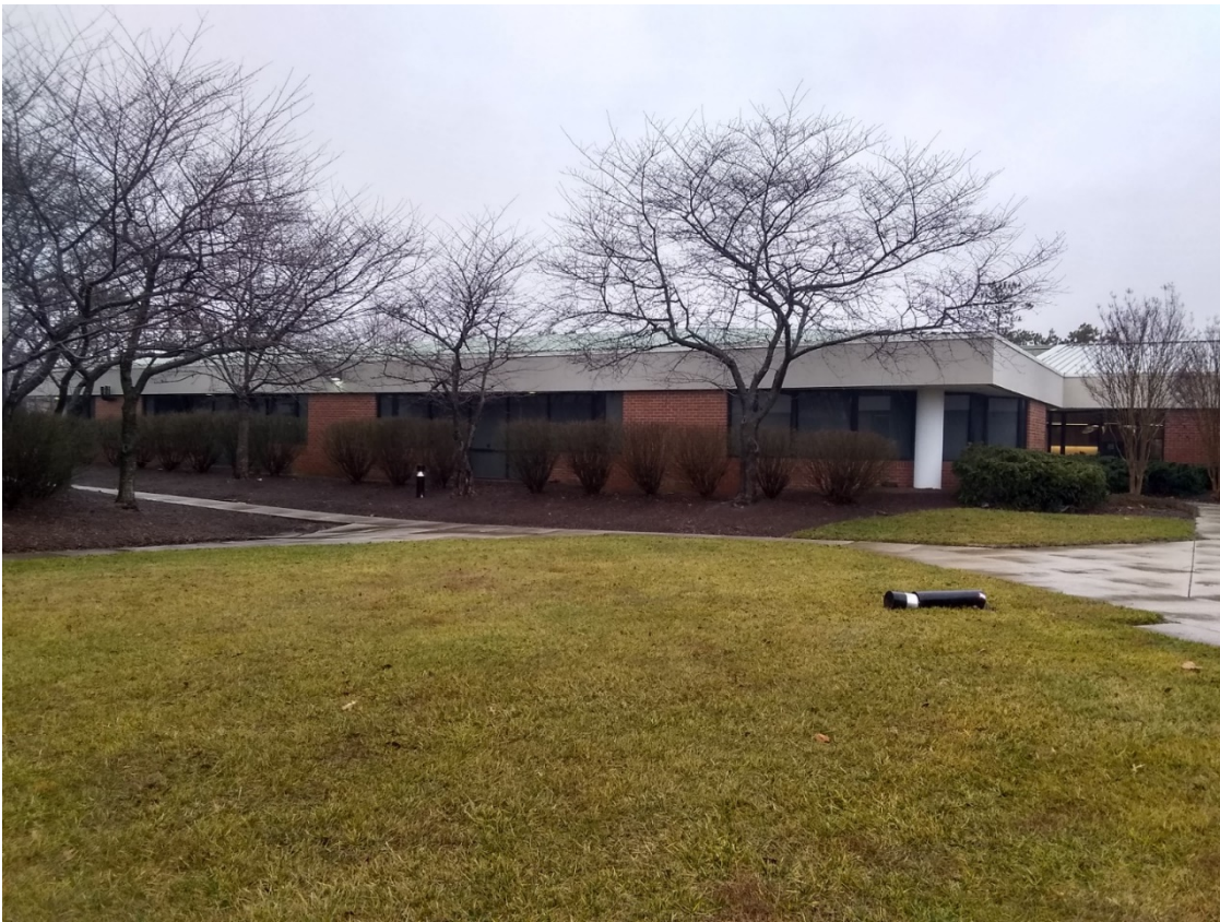
VIEW LOOKING NORTHWEST AT BUILDING EAST ELEVATION
