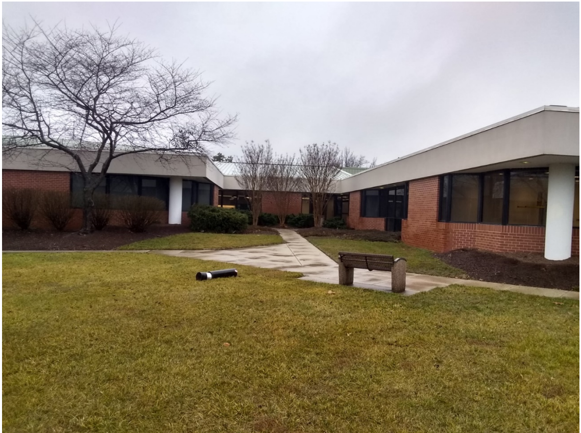
VIEW LOOKING NORTHWEST AT BUILDING EAST ELEVATION
