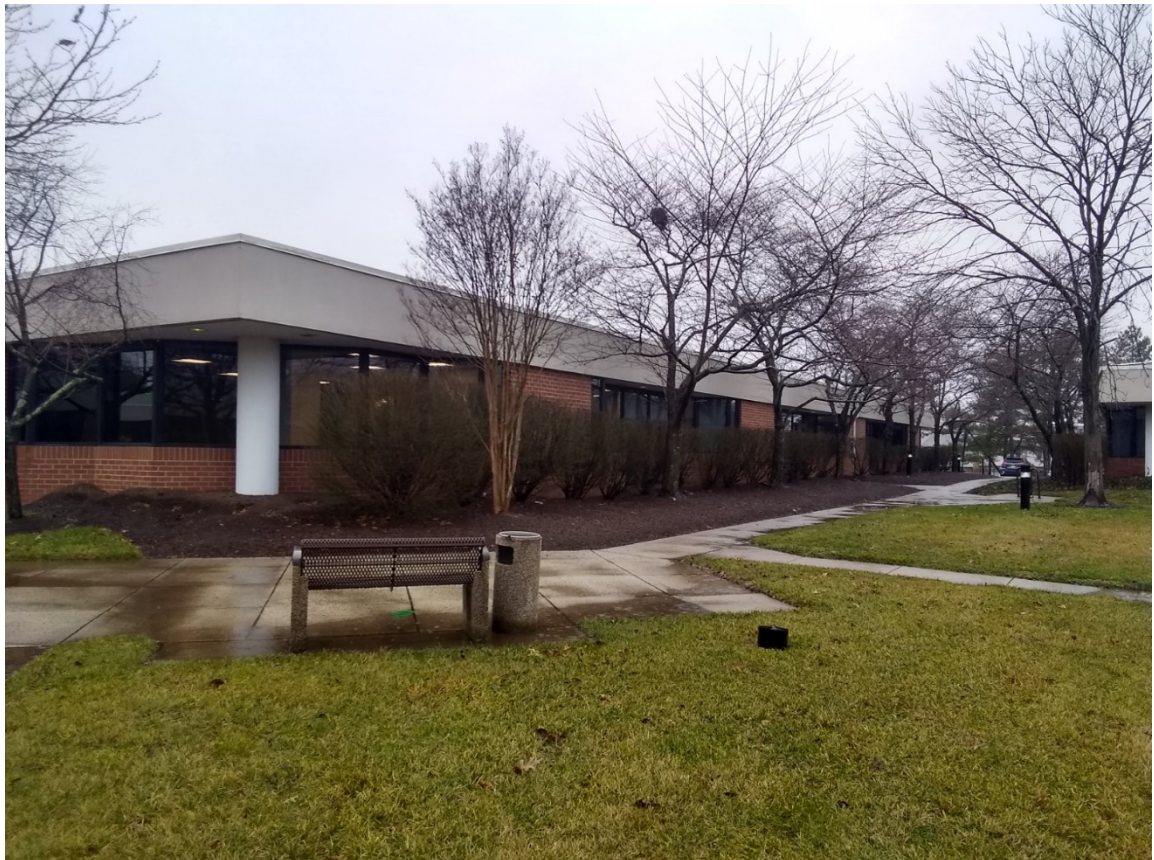
VIEW LOOKING SOUTHWEST AT BUILDING NORTH ELEVATION
