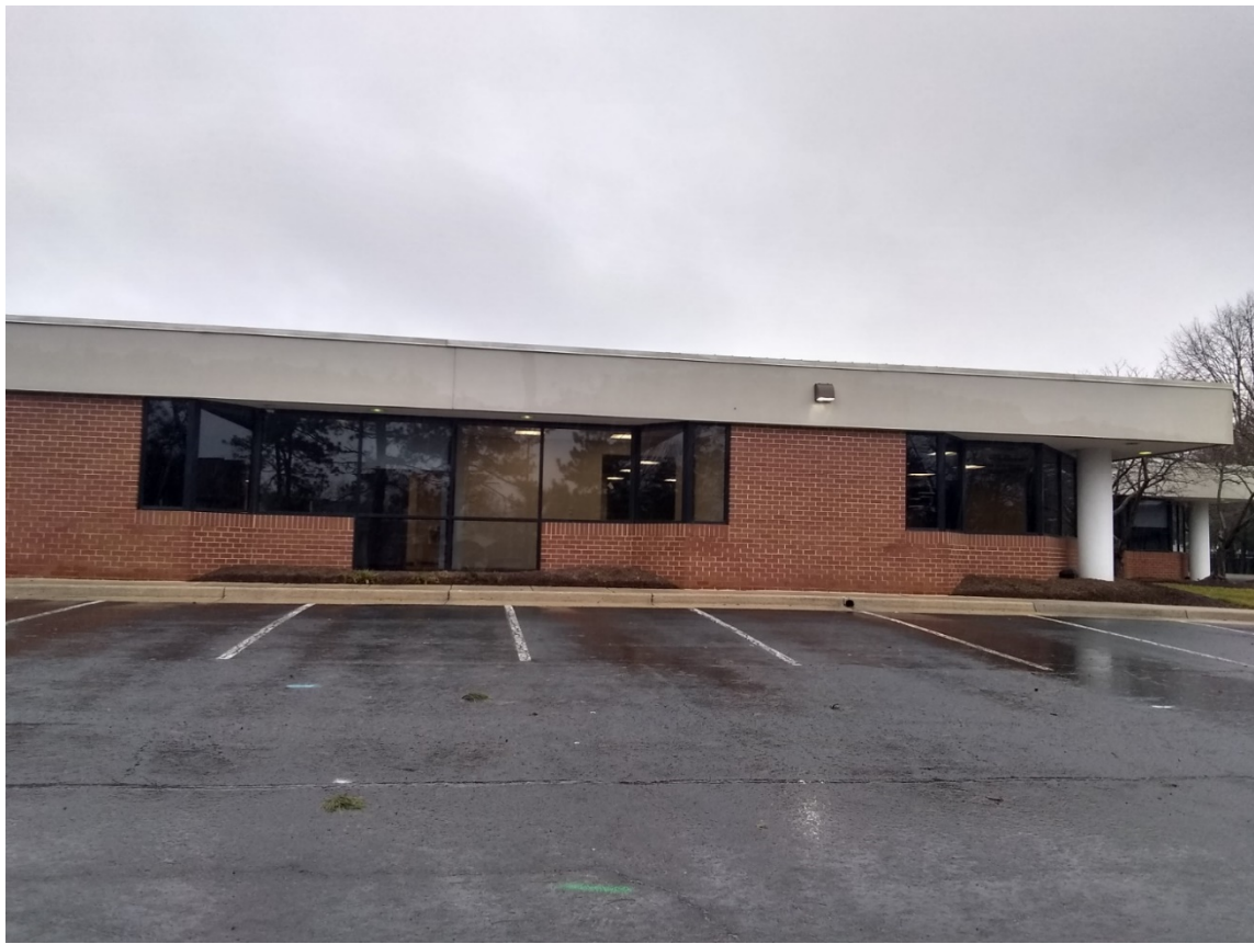
VIEW LOOKING SOUTHEAST AT BUILDING WEST ELEVATION
