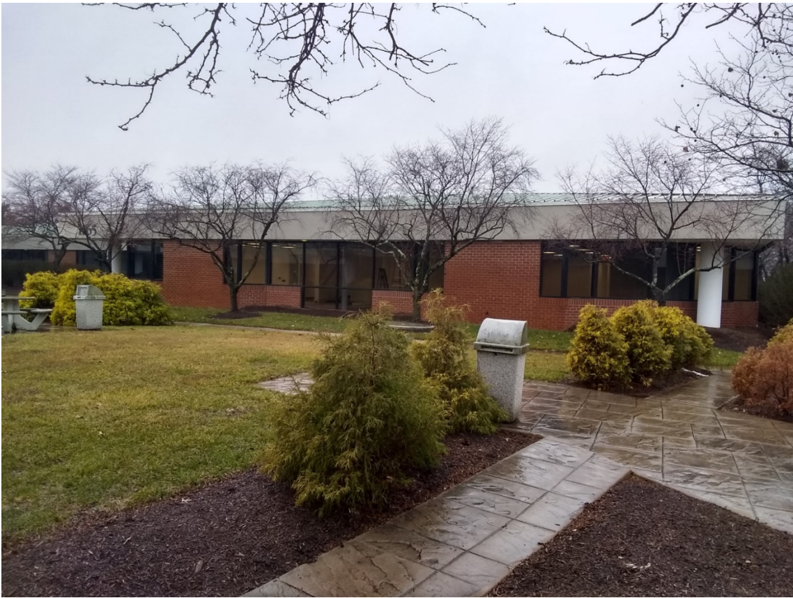
VIEW LOOKING SOUTHWEST AT BUILDING EAST ELEVATION
