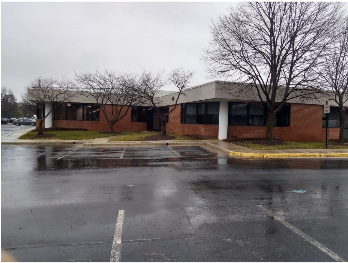
VIEW LOOKING NORTHEAST AT BUILDING SOUTH ELEVATION
