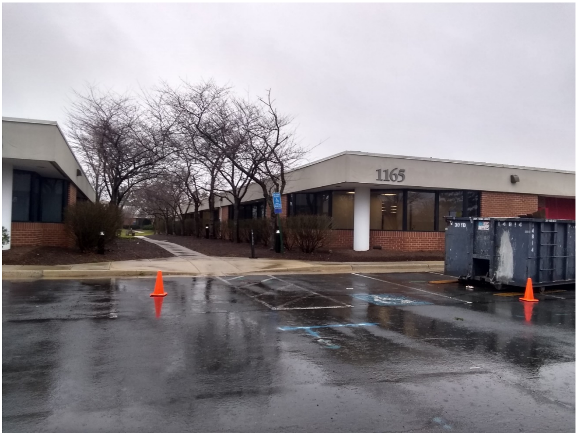
VIEW LOOKING SOUTHEAST AT BUILDING NORTH ELEVATION
