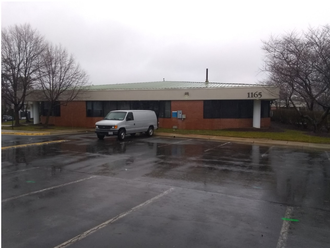
VIEW LOOKING NORTHEAST AT BUILDING SOUTH ELEVATION
