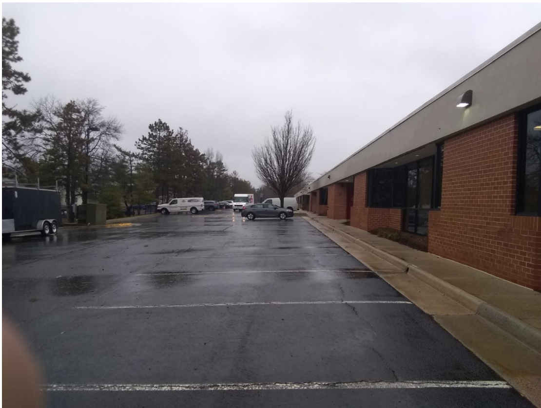
VIEW LOOKING NORTHEAST ALONG WEST BUILDING ELEVATION
