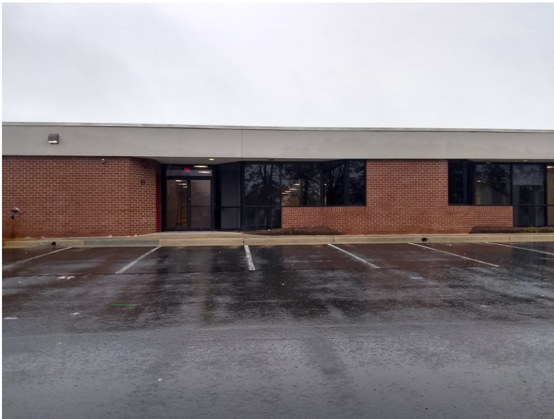
VIEW LOOKING SOUTHEAST AT PLANNED GENERATOR LOCATION
