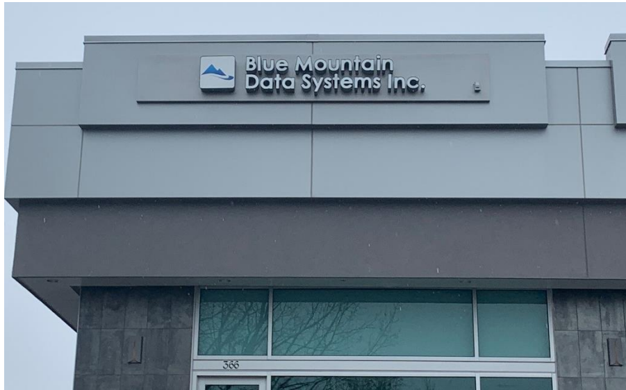
Exhibit 2: Staff photo of existing conditions on the northeast corner of 311 Spring St. and end tenant space dated 02/11/2020
