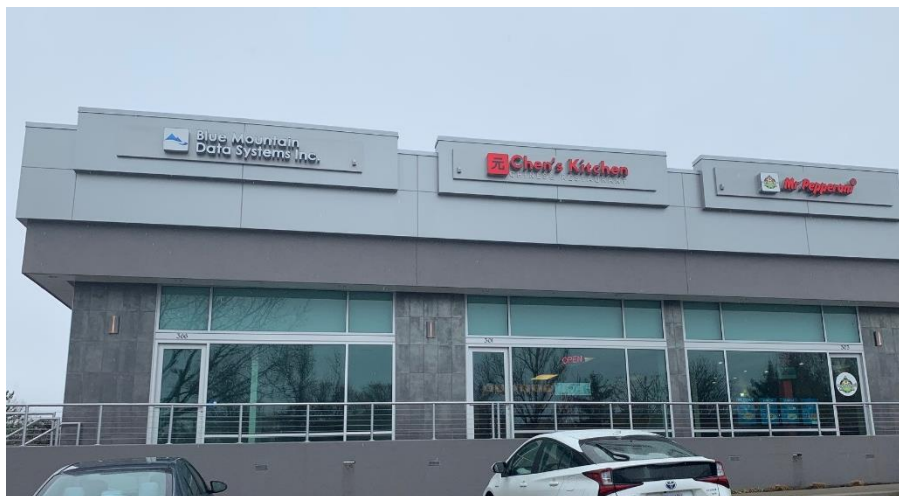
Exhibit 1: Staff photo of existing conditions on the northeast corner of 311 Spring St. dated 02/11/2020
