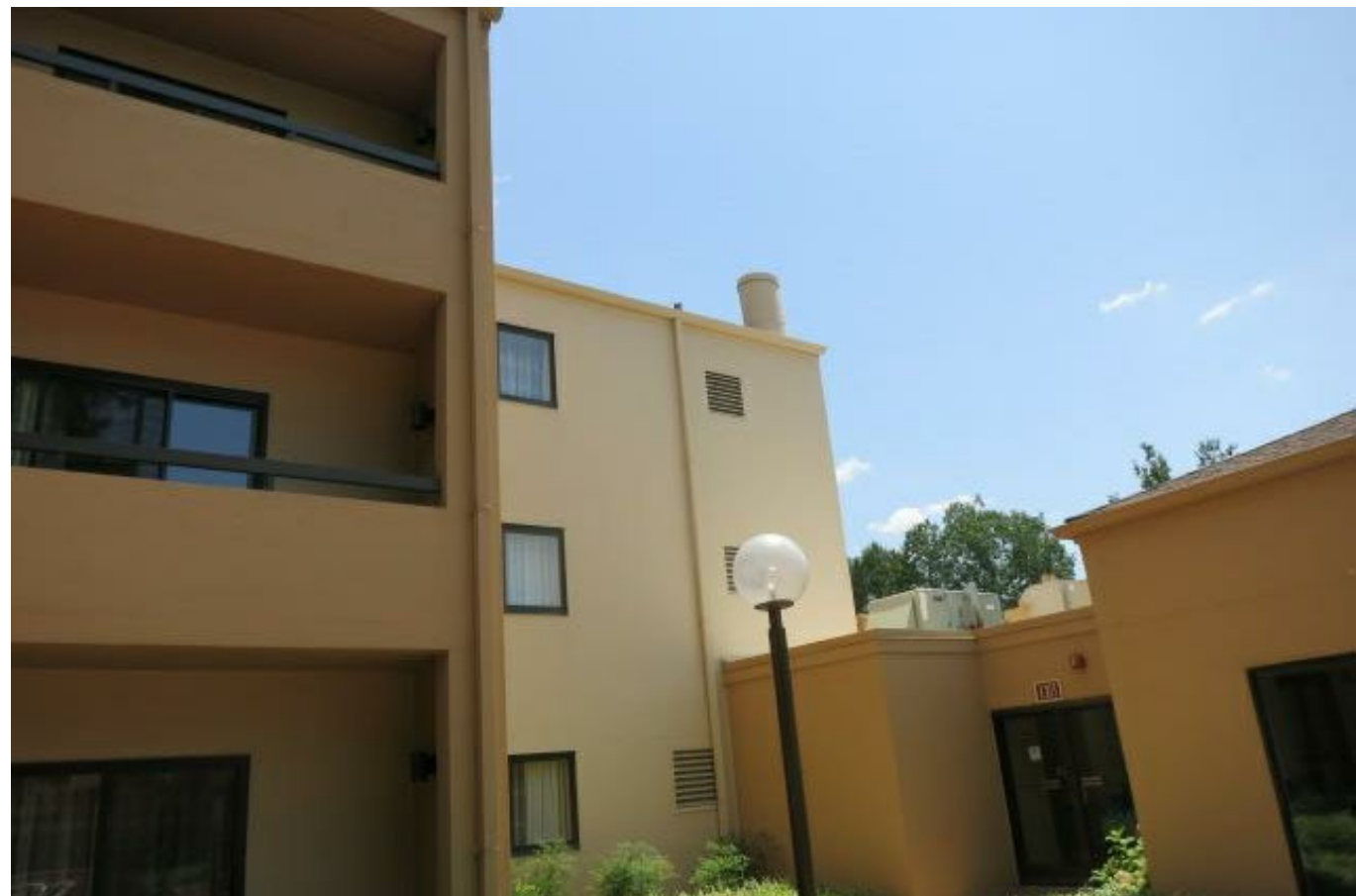
1 EXTERIOR PHOTOS - EAST COURTYARD 3/32" = 1'-0"
