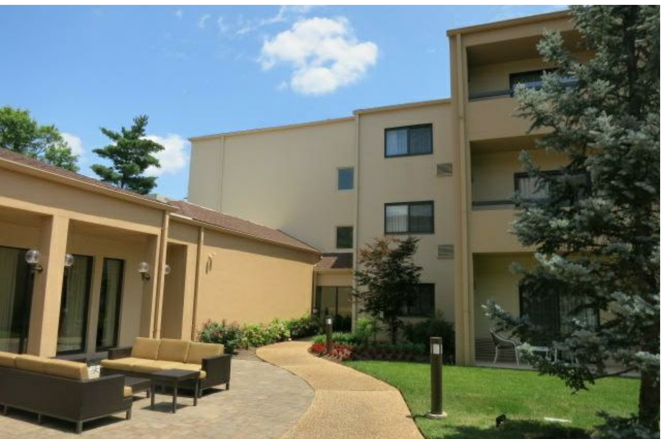
2 EXTERIOR PHOTOS - NORTH COURTYARD 3/32" = 1'-0"
