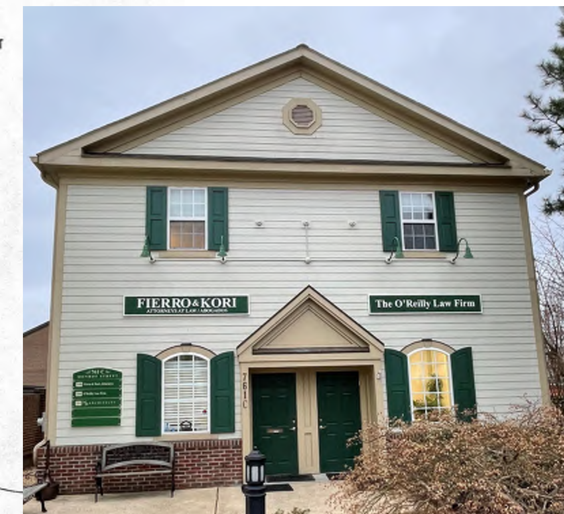
EXISTING PICTURE OF 761C
