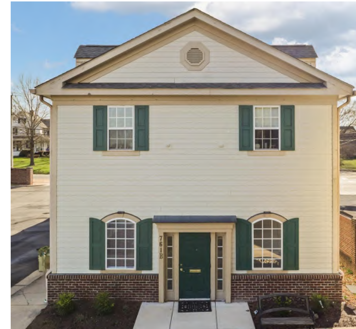
EXISTING PICTURE OF 761B
