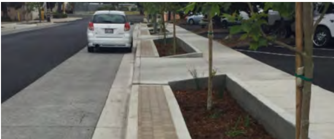
Pervious paving at on-street parking, pervious pavers at step-out zone, and narrow rain garden on sidewalk
