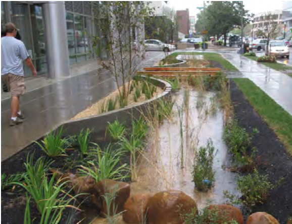
Bioretention bioswale on sidewalk, Baltimore, MD
