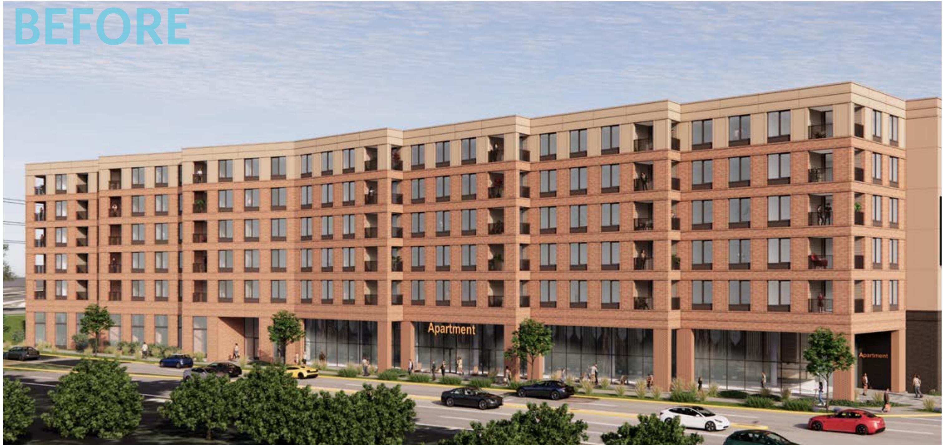
HERDON PARKWAY FACADE
