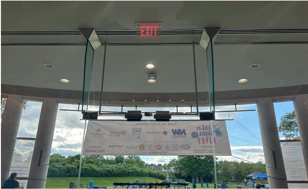
West Elevation - Interior Storefront System and Details, May 2025
