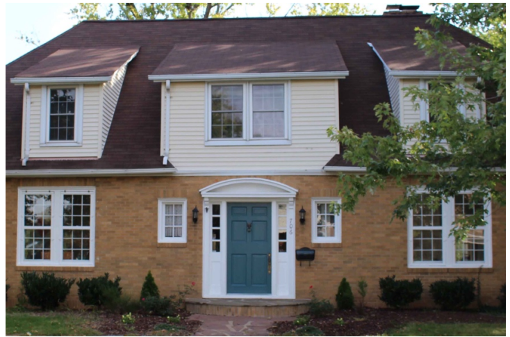
Photograph - Secondary Elevations or Details
