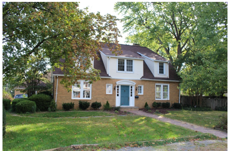
Photograph - Primary Elevation(s)
