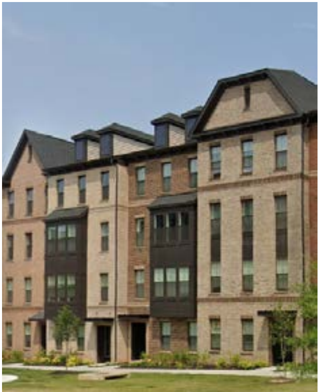
Outside corner brick wrap and transition a different color brick at an inside corner
