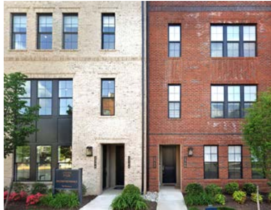
Brick banding; materials color changes; style appropriate trim; matching mortar vs contrasting mortar; unified metal color
