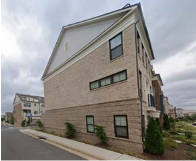
Brick rowlock band and color change make a transition defining the Base from the Body; brick at Base is patterned; brick at Body is typical running bond with matching mortar
