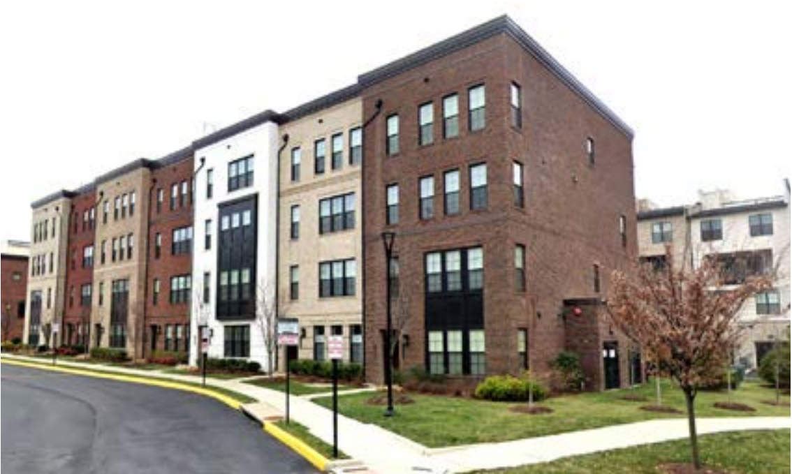
FLAT ROOF with PARAPET Shed style roof is concealed by the parapet at front & side (shed at back is exposed)
