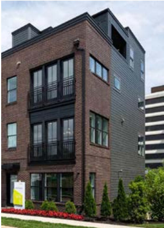
Outside corner brick wrap and transition to siding
