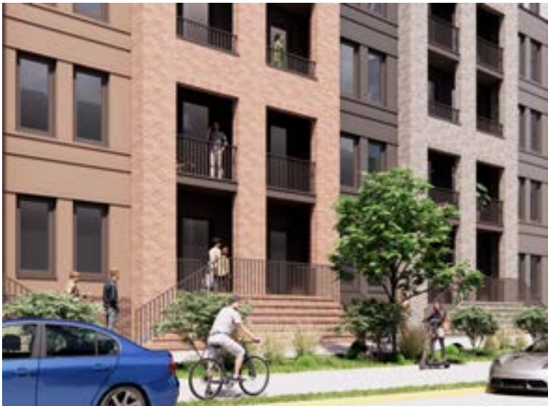
ARTICULATION AT THE STREET LEVEL Articulated Individual Residential Stoops & Foundation Plantings
