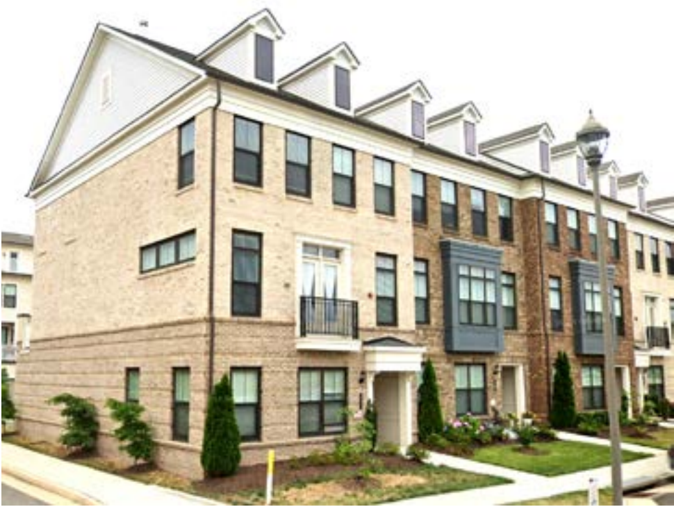
SINGLE GABLE ROOF Uniform roof line is emphasized by cornice trim at eaves
