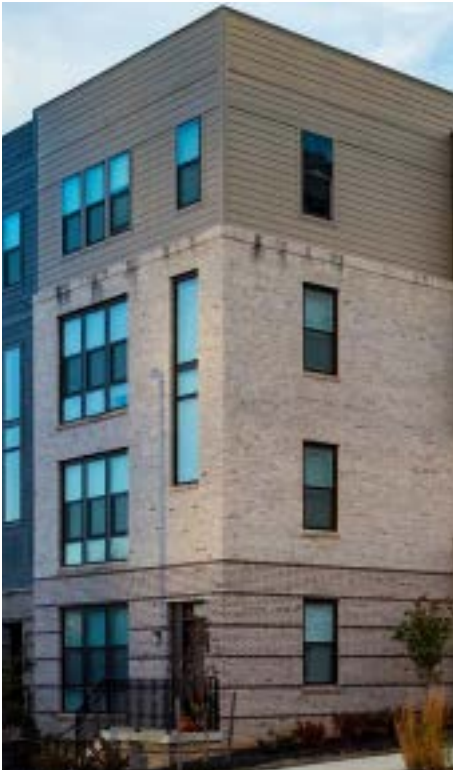
Outside corner brick and siding wrap at end facade
