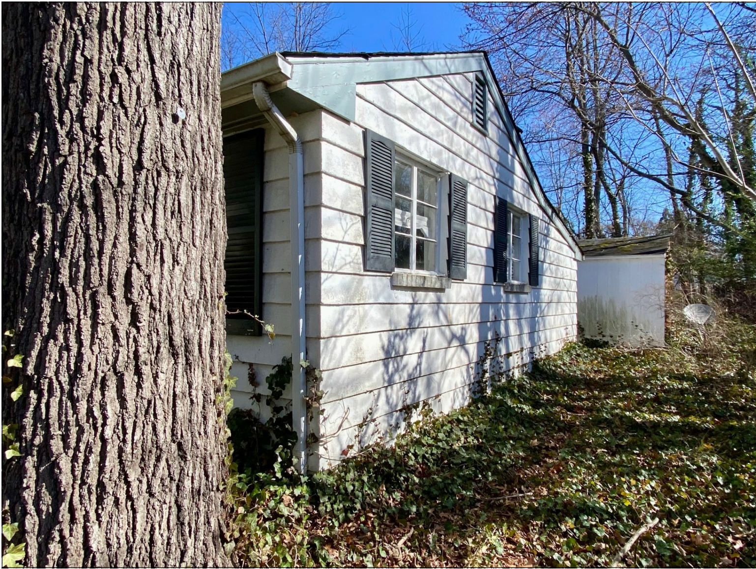
EXISTING GRADE AT FRONT RIGHT CORNER
