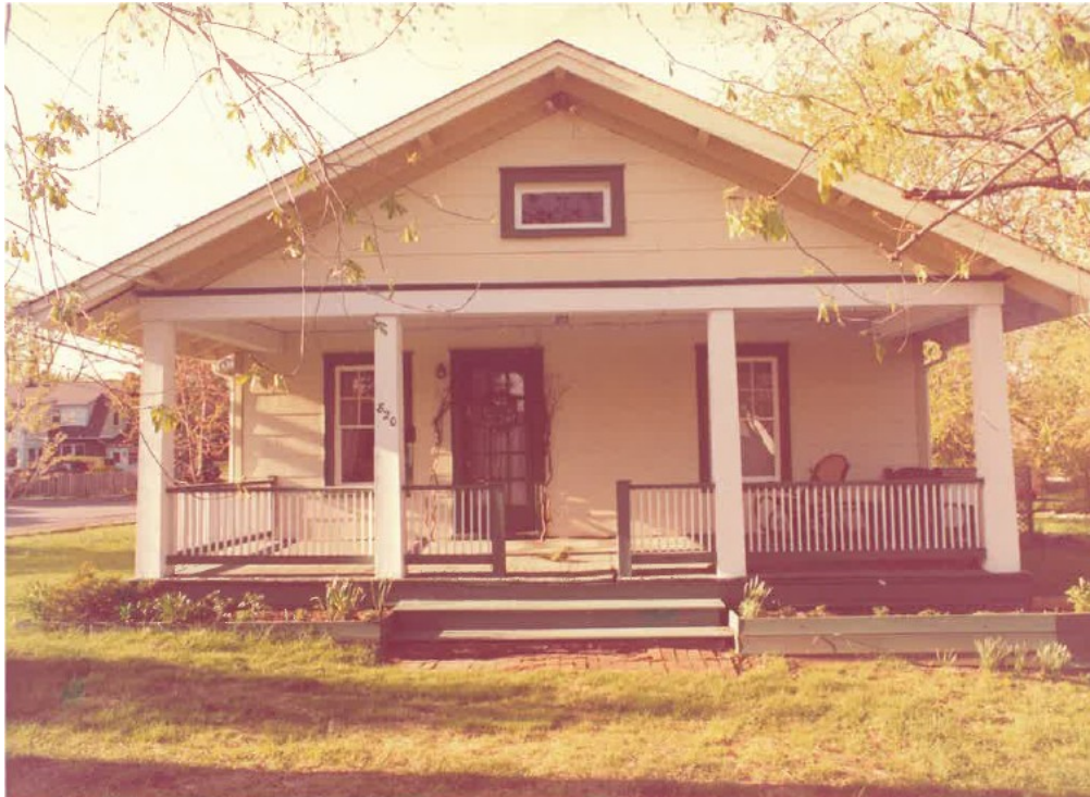
Figure 2: Façade (South Elevation) prior to second floor addition completed according to HPRB 97-7, 1997. Note the alteration to the front porch that occurred between 1987 and 1997.
