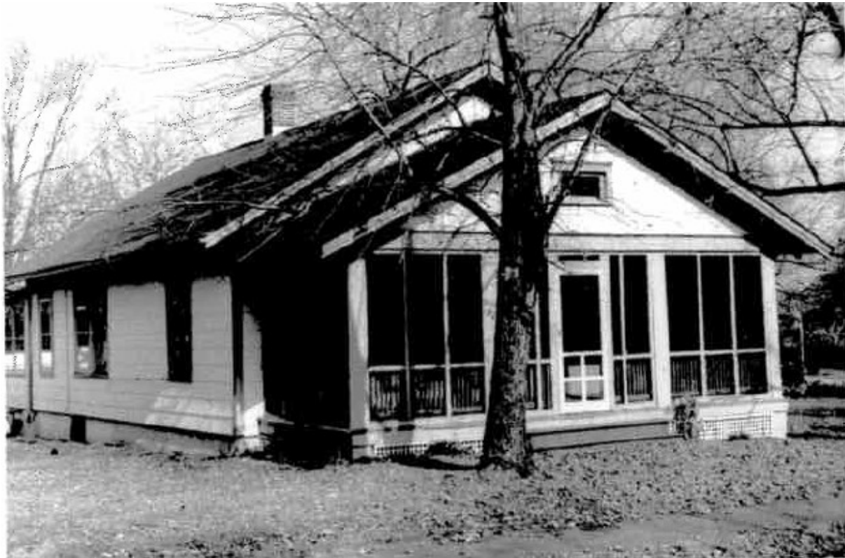
Figure 1: 1987 architectural survey photograph showing the porch prior to circa 1998 alteration. Source: Town of Herndon
