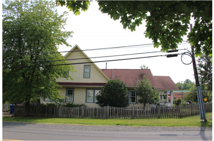
Photograph - Secondary Elevations or Details
