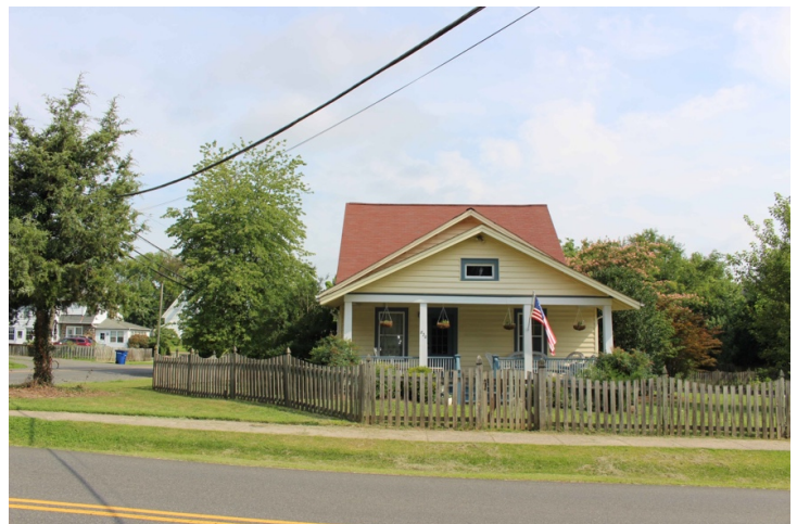
Photograph - Primary Elevation(s)
