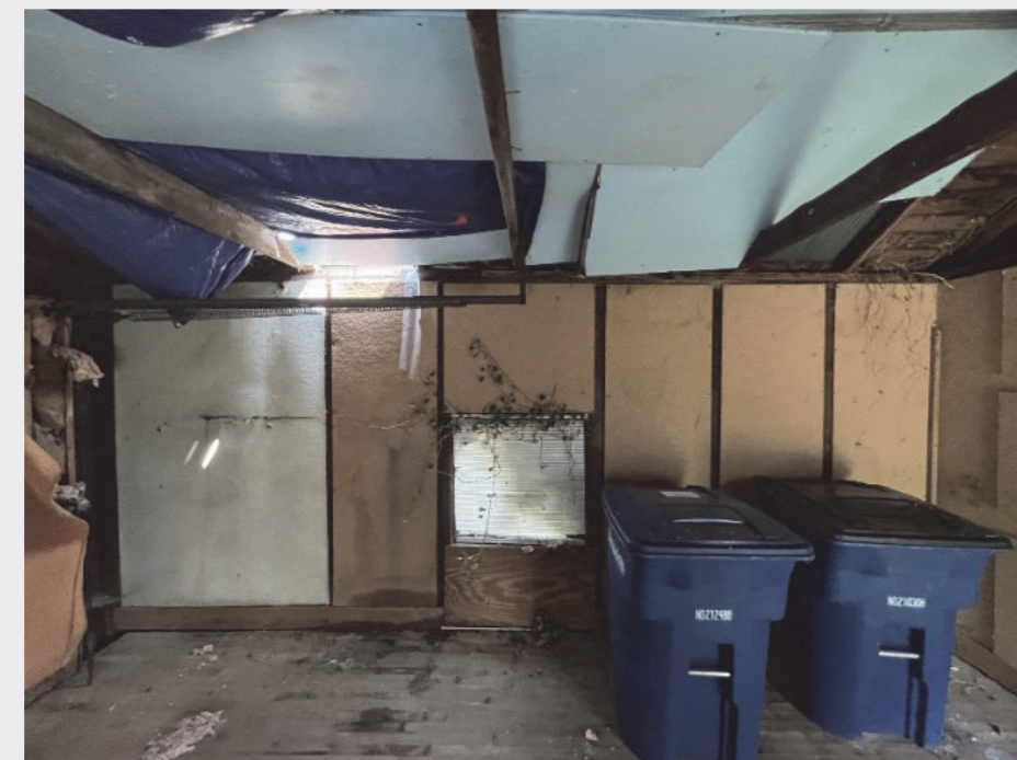
GARAGE INTERIOR (LOOKING TOWARD LONG SIDE)
