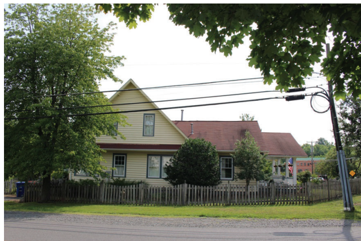
Photograph - Secondary Elevations or Details
