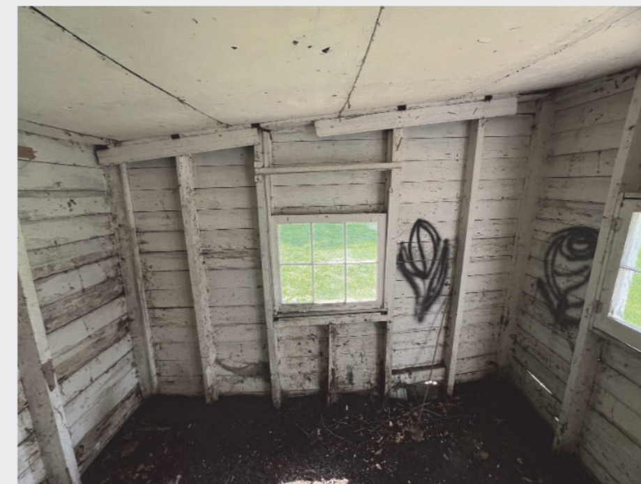
SHED INTERIOR (LOOKING TOWARD REAR)
