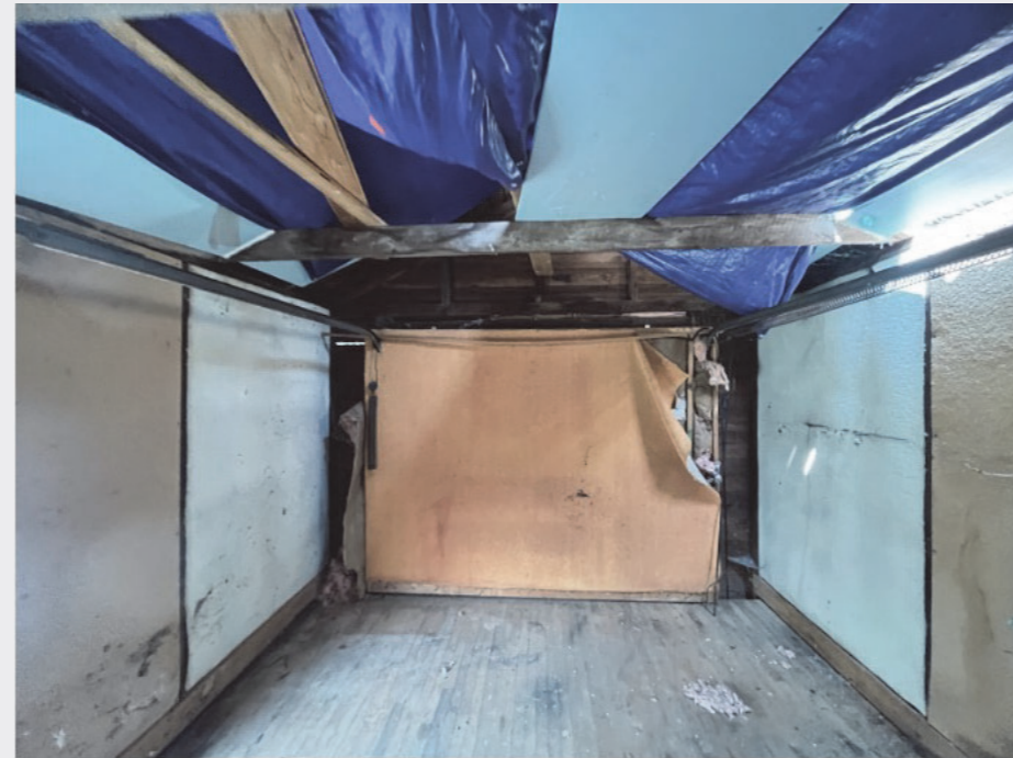
GARAGE INTERIOR (LOOKING TOWARD GARAGE DOOR)
