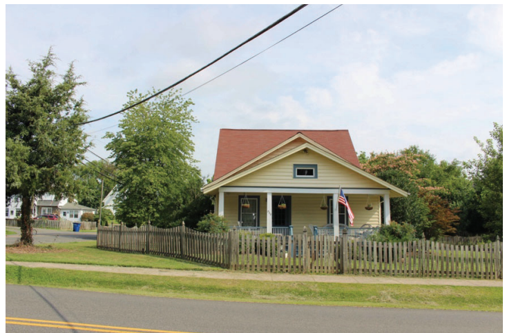
Photograph - Primary Elevation(s)
