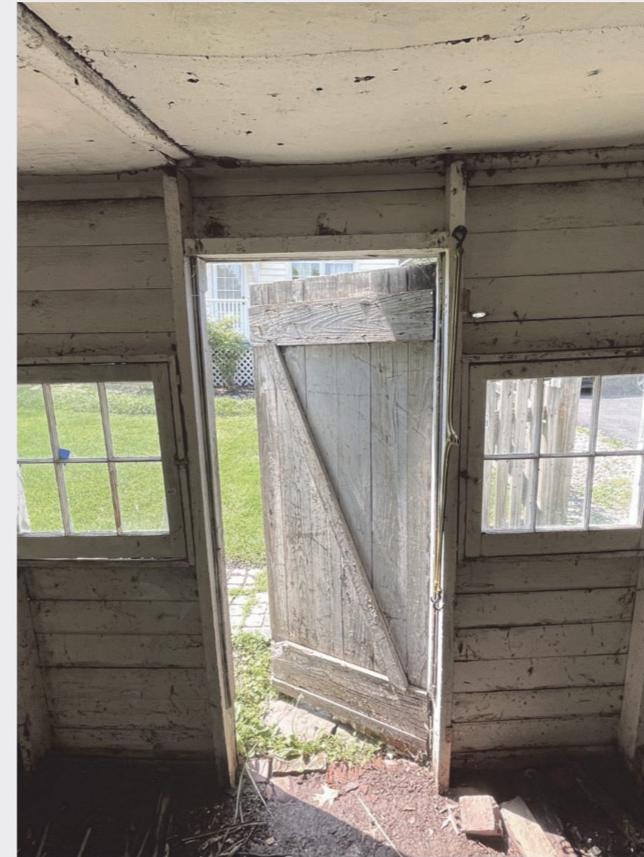
SHED INTERIOR (LOOKING TOWARD DOOR)
