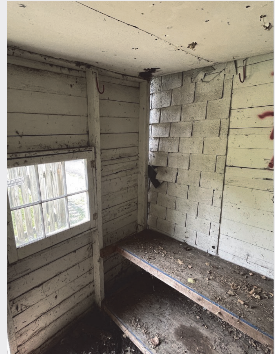
SHED INTERIOR (LOOKING TOWARD SIDE CORNER)
