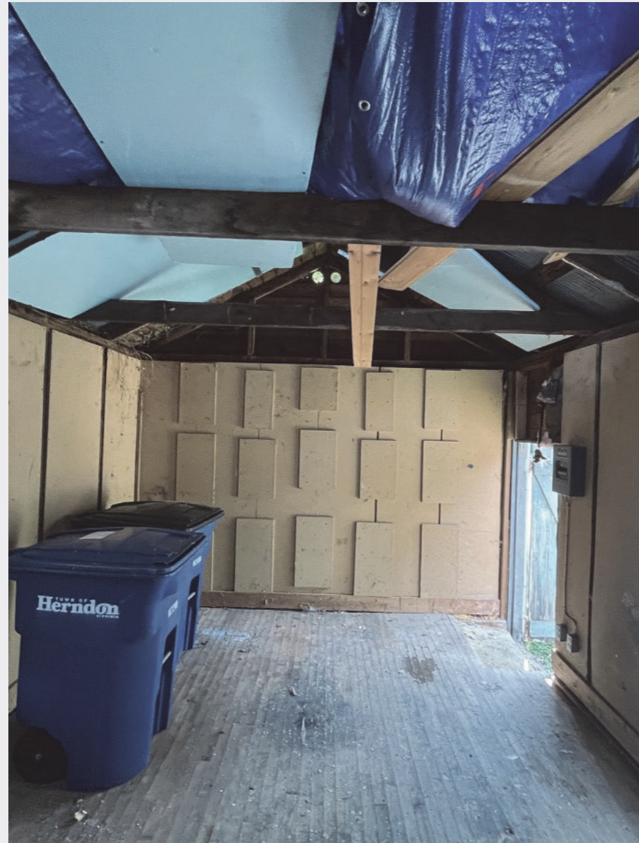
GARAGE INTERIOR (LOOKING TOWARD SHED ADDITION)
