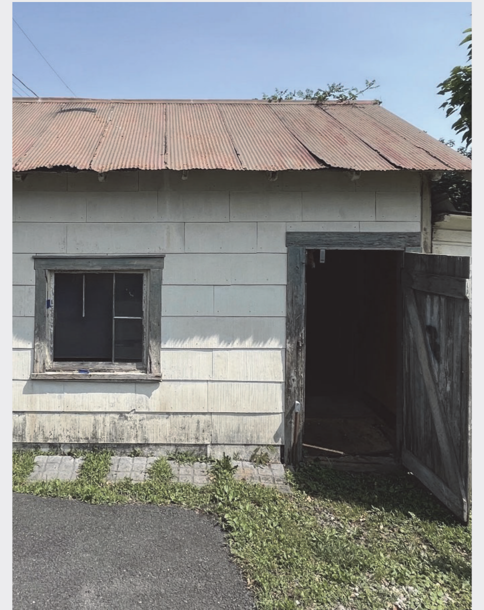
CLOSE UP OF CLADDING, DOOR & WINDOW
