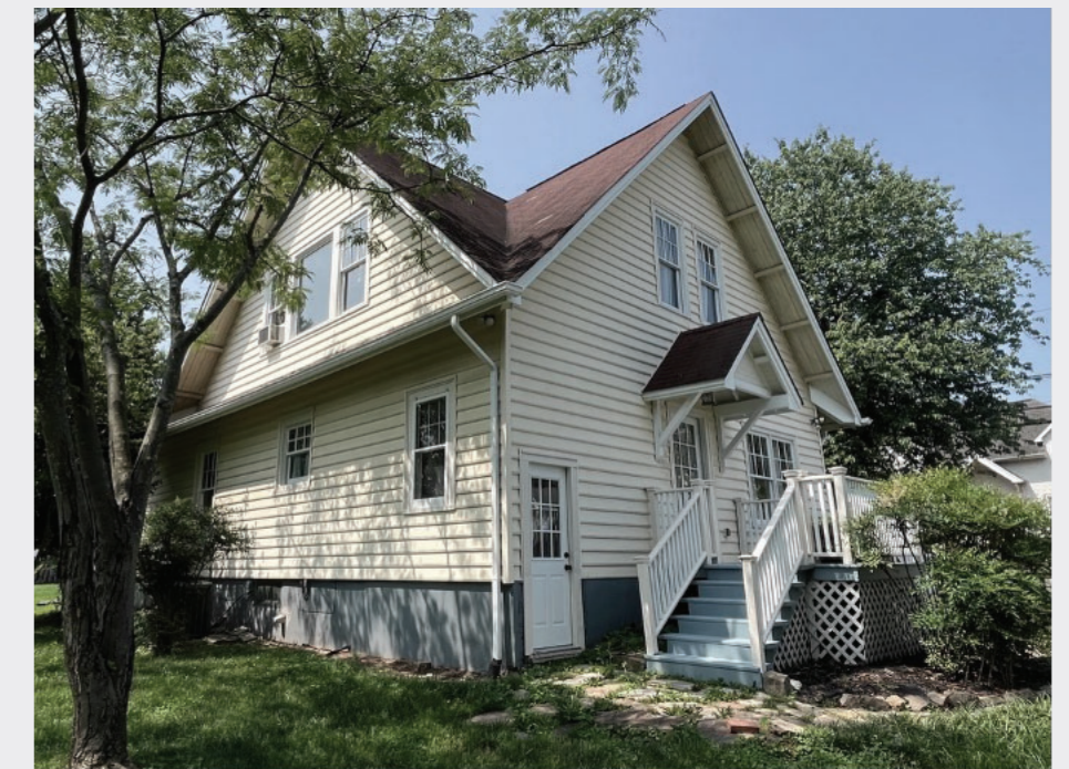
REAR / SIDE CORNER
