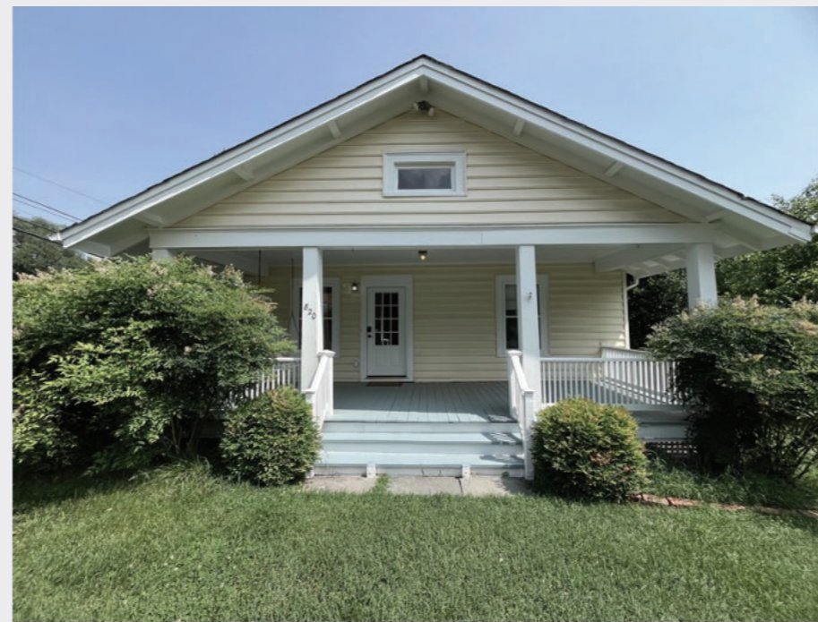
FRONT PORCH (LOCUST STREET ELEVATION)
