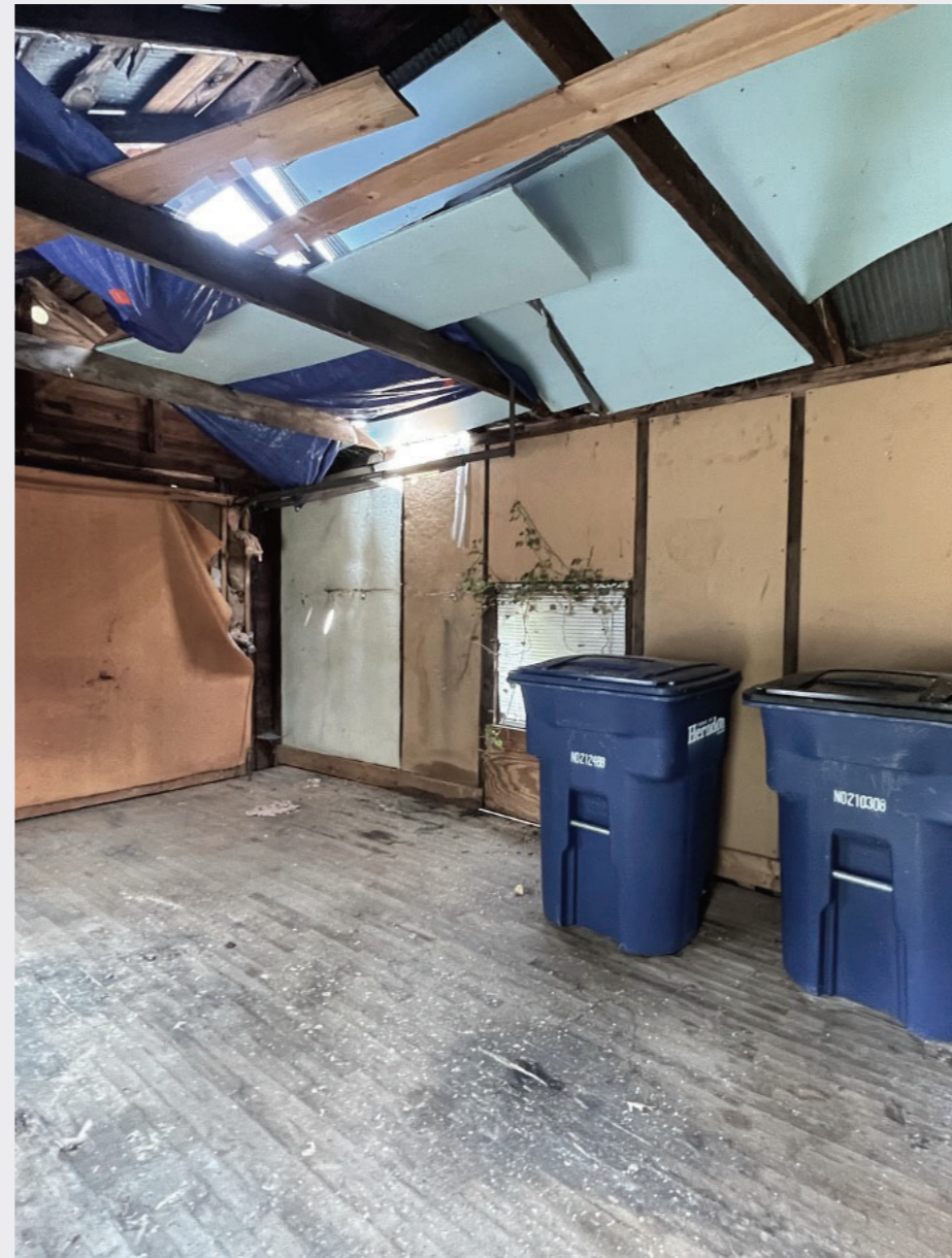
GARAGE INTERIOR (LOOKING TOWARD FRONT CORNER)
