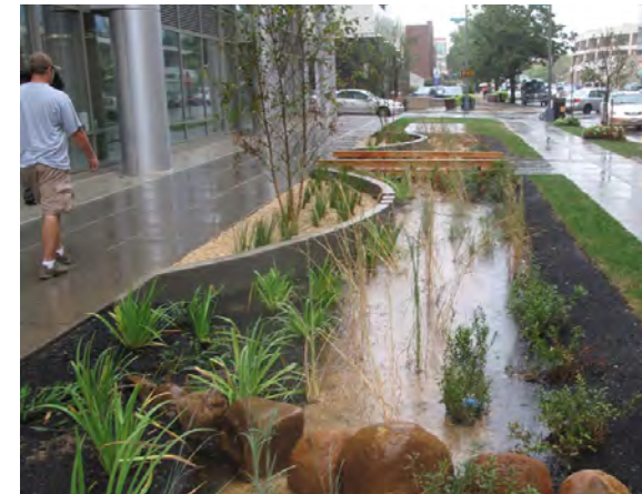
Bioretention bioswale on sidewalk, Baltimore, MD
