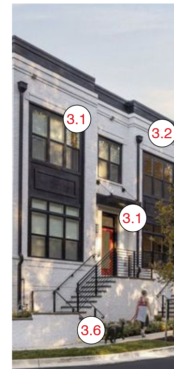
Example of a 2 story bay window & recessed window groupings - with decorative metal surround and with siding surrounds; materials defined by color - (1) brick color & (1) color for all decorative metal
