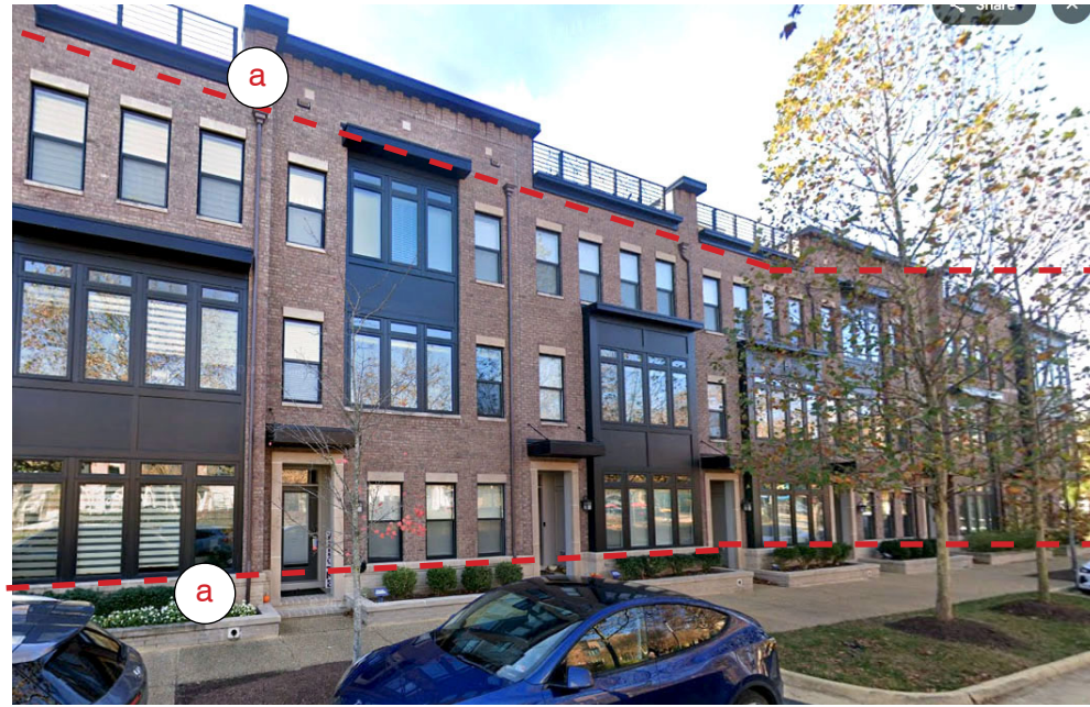
VERTICAL DIVISIONS WITH A SMALL BASE & TOP A monochrome brick & mortar color for the large body portion of the facade; material changes indicate the smaller cast stone base and the metal cornice “cap”
