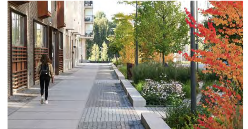
Pervious pavers demarcating entryways and pedestrian circulation next to fully grown rain garden
