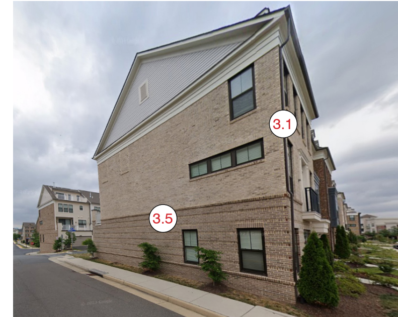
All materials turn the outside corner and extend at least 2ft or 2ft beyond openings; horizontal transition is extended at least 2ft above the openings
