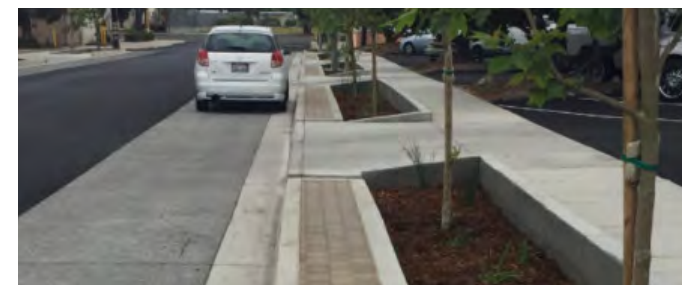
Pervious paving at on-street parking, pervious pavers at step-out zone, and narrow rain garden on sidewalk
