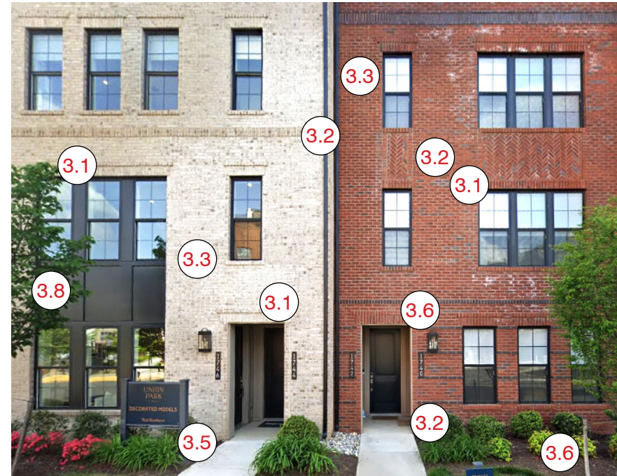
Architectural features - window grouping, recessed entry. Enhanced brick detailing - pulled brick band, decorative brick pattern, alternating color brick coursing. No expanse of brick greater than 10FT. Entry framed by planting zone
