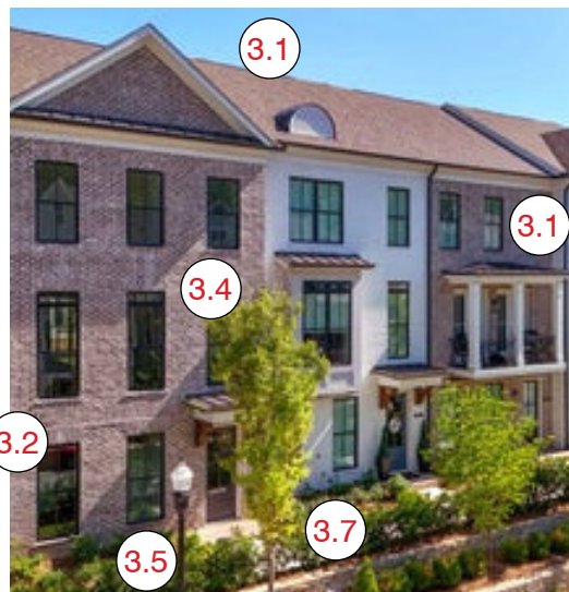
3.0 Dormers; patio doors with balcony; covered entry; front facing secondary gable; single story bay (For two story bays, see examples on this page and on pg 10)
