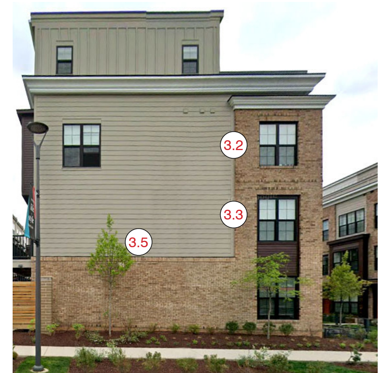
3.2 Outside corner brick wrap and transition to siding
