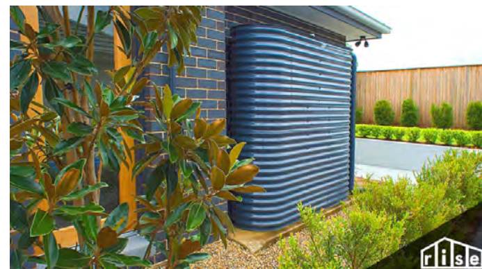
Rainwater harvesting cistern
