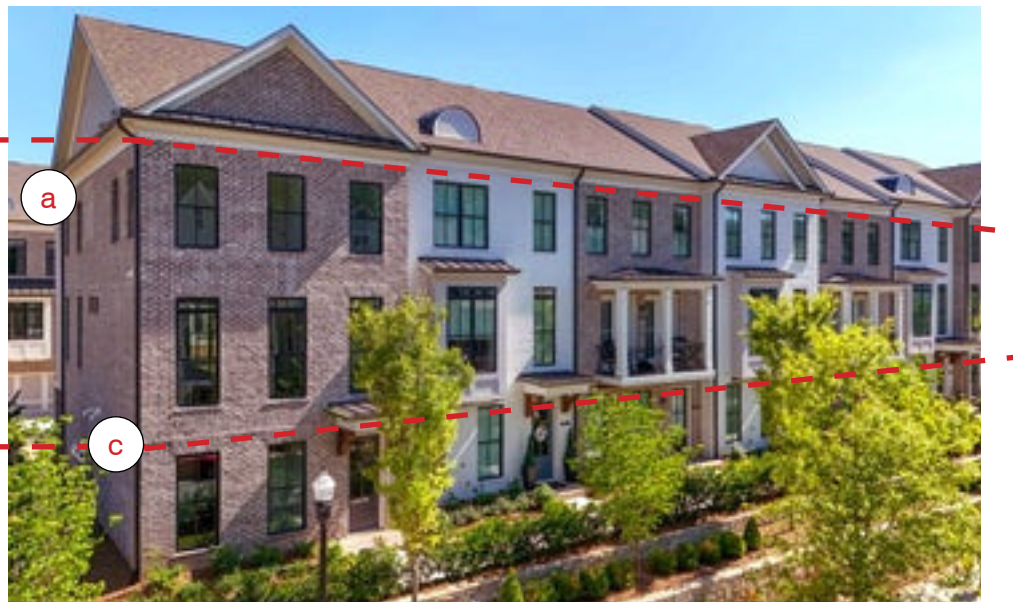
VERTICAL DIVISIONS WITH BELT COURSES IN MONOCHROME BRICK A single brick & mortar color; simple belt coursing indicate section changes
