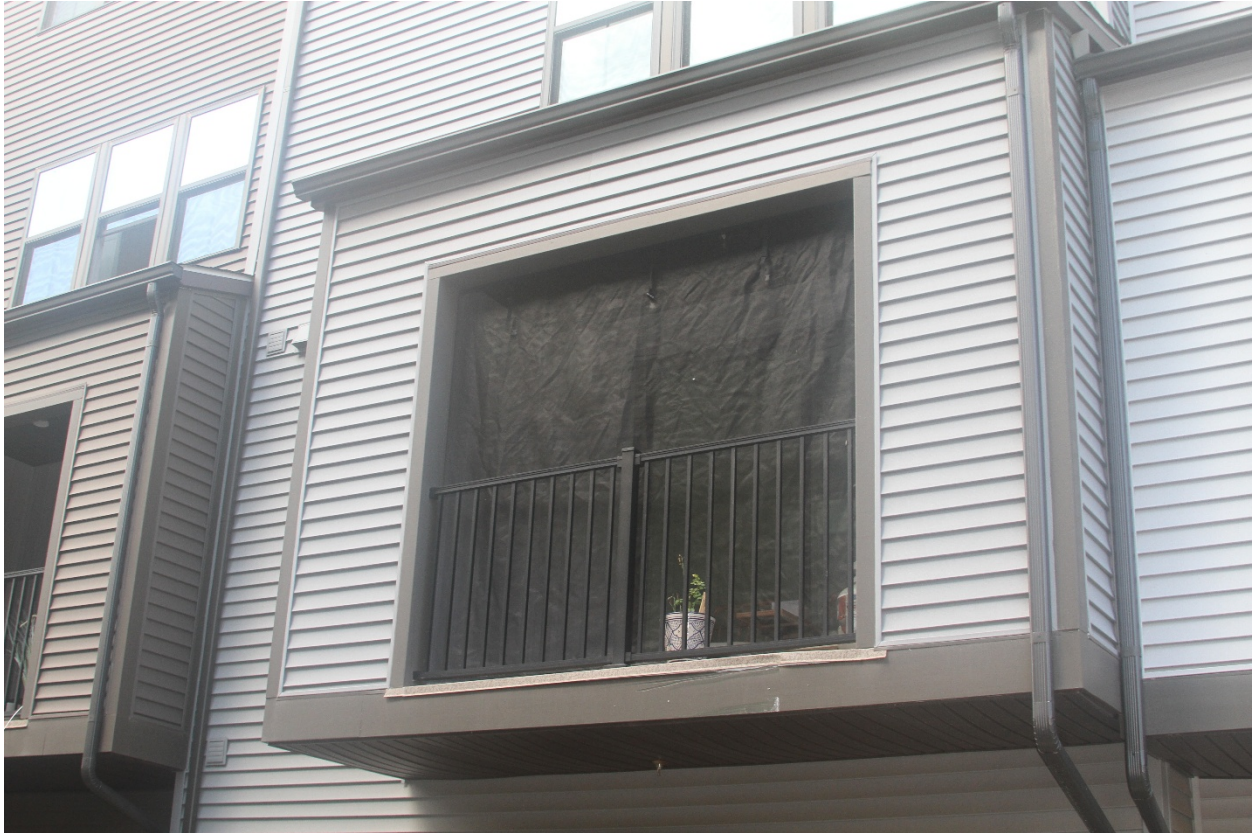
Figure 5: Example of an inset balcony from Woodland Park development.
