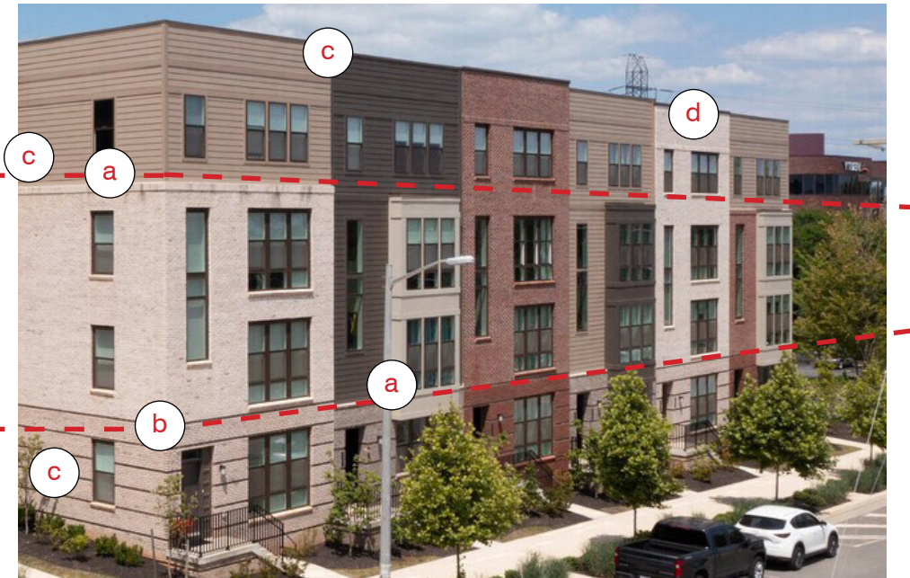
VERTICAL DIVISIONS WITH COLOR & COURSING CONTRASTS Two masonry colors with different coursing separate the base from the body; the top is indicated by the cornice on the front but includes the roof at the end condition
