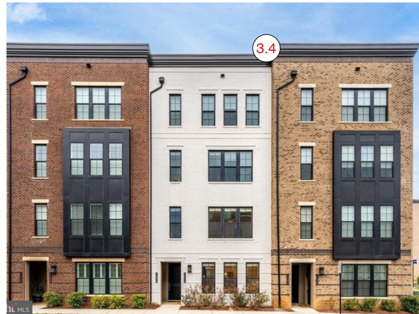
All materials turn the outside corner and extend at least 2ft or 2ft beyond openings; horizontal transition is extended at least 2ft above the openings
