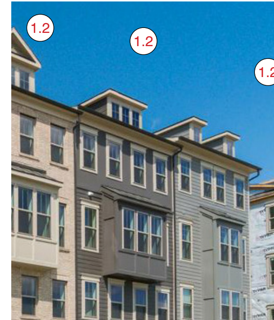
1.2 MAIN GABLED ROOF w/ DORMERS Gabled dormer shown on left; two types of hipped dormers on the right
