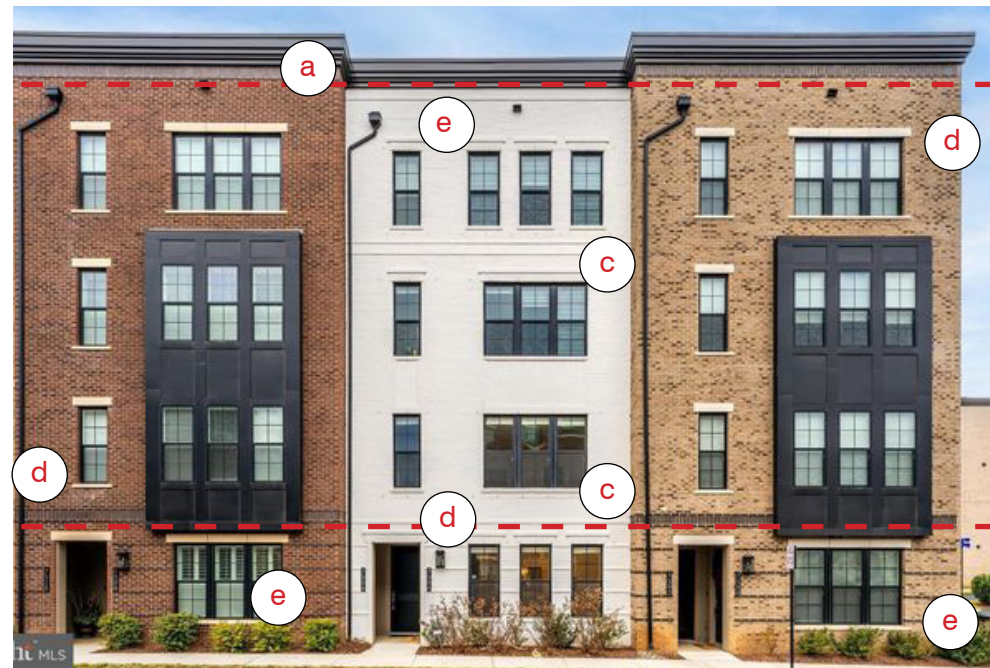
VERTICAL DIVISIONS WITH MONOCHROME UNIT ELEVATIONS A single brick & mortar color per unit; contrasting colors and brick coursing indicate the base while material changes indicate the “cap”
