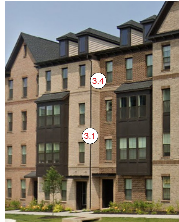
3.1 Outside corner brick wrap and transition a different color brick at an inside corner
