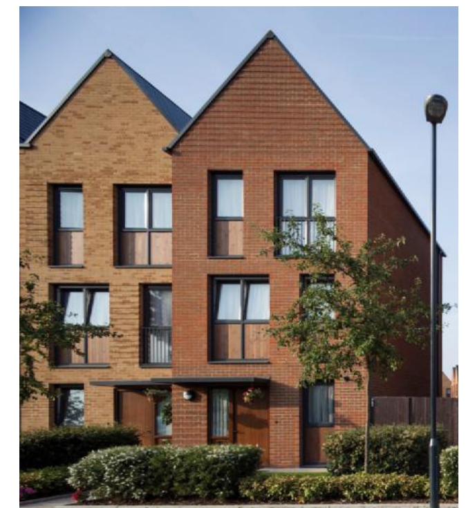
1.d INDIVIDUAL FRONT FACING GABLES Used here along with changes in facade color to emphasize and identify individual units
